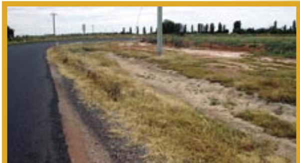
Compaction during road and house construction may impact on the lateral flow of water. Salt crystals and salinity tolerant vegetation beside the road, as in this photo, may indicate this process.
