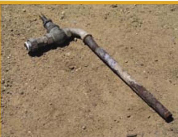
Metal pipes, taps, tanks and fences rust quicker in a saline environment. Permeable cement also allows salty water to penetrate so that the reinforcing steel within the cement rusts. Over time the strength given to the cement by the reinforcing is diminished.
