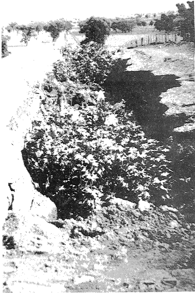
Figure 1 Severe gully erosion has undercut the road pavement on Cooramin Street - Cartwright's Hill, following a high intensity storm in March, 1966.
