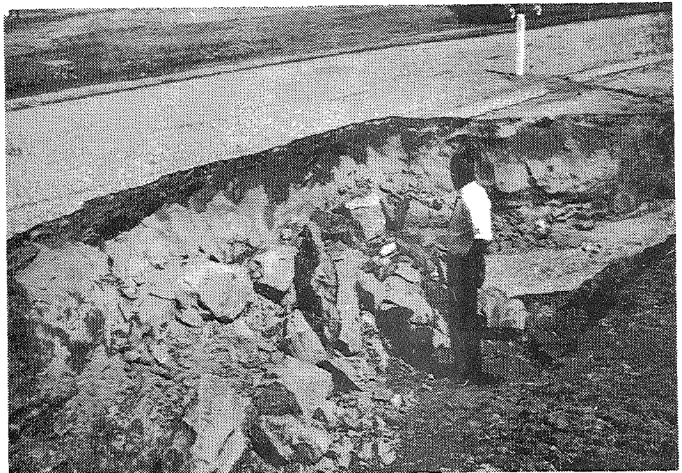
Figure 1 Severe gully erosion has undercut the road pavement on Cooramin Street - Cartwright's Hill, following a high intensity storm in March, 1966.
