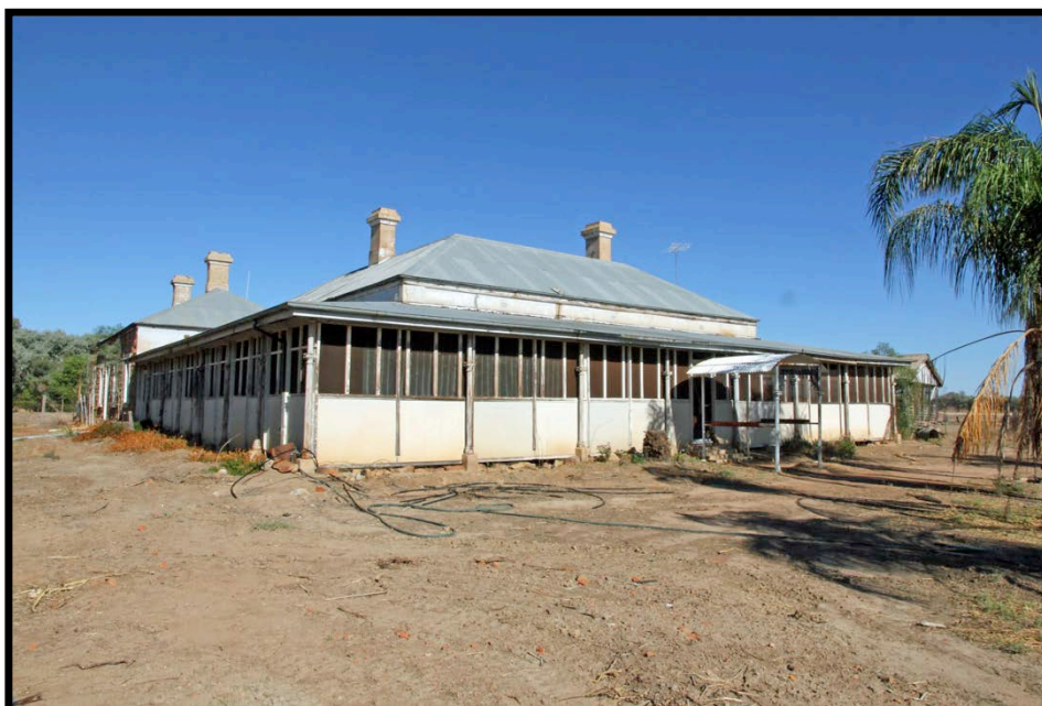
Figure 3.8 Dunlop Homestead today photographed from approximately the same angle. Photograph by Sheppard April 2013.
