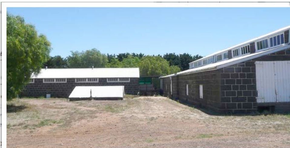
Figure 3.19 Some of the fine sheds at Titanga Station with dressed coursed Basalt blockwork. Courtesy www.onmydoorstep.cm.au/heritage-listing .
