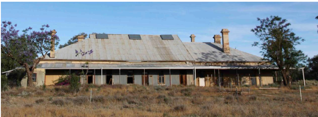
Figure 3.1: The Toorale Homestead west elevation. Photograph by Sheppard 2012.
