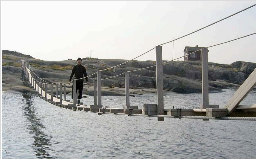
Above: Soderskar bridge, Finland, a very simple, long and narrow suspension bridge. (Image courtesy Wikipedia Commons, Miika Silverberg September, 2005)
