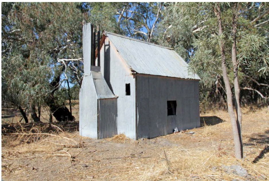
Figure 8.5: The Chinese gardeners Hut at Dunlop Station, which was probably the same as, or very similar to the Toorale Chinese gardeners Hut. (Photograph by Sheppard, April 2013.)
