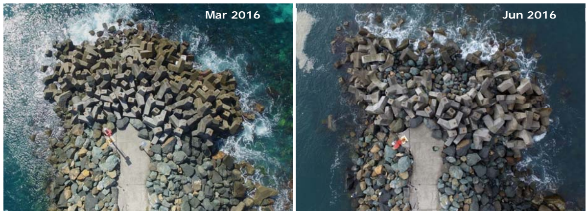
Figure 4.6. Forster breakwater head before and after June 2016 storm. Source: Crown Lands
