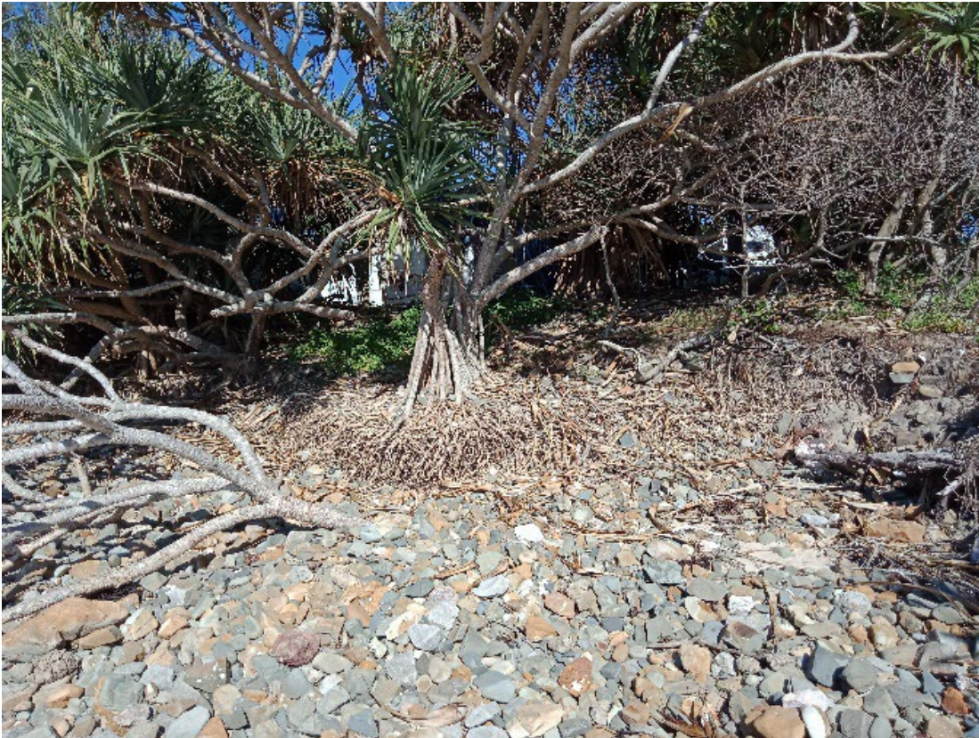
Photo 9 Riverbank erosion occurring 10 metres south of access stairs, Sandon River campground, 2023
