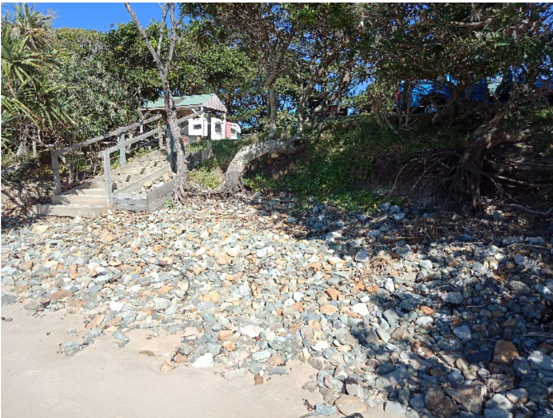
Photo 10 Riverbank erosion occurring immediately north of access stairs, Sandon River campground, 2023
