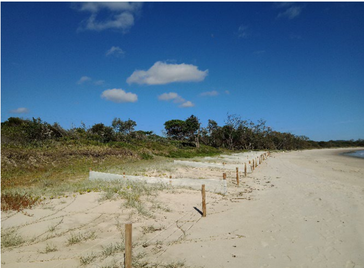
Photo 4 Dune rehabilitation area adjacent to Sandon River campground, 2023
