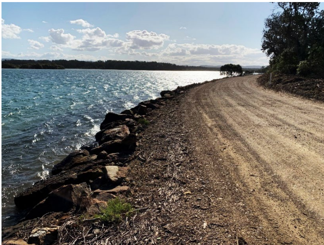
Photo 5 Section of Sandon River Road armoured with rock protection, 2020
