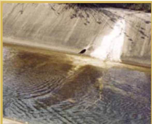
Clear water in a stormwater channel. Photo: DIPNR
