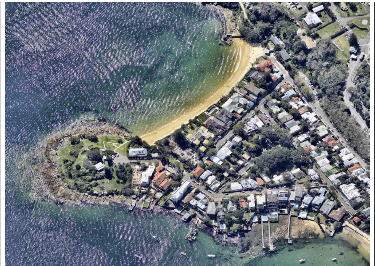
Figure 7 – Aerial photograph of the South Head, Camp Cove and Green Point Precinct Source: nearmap
