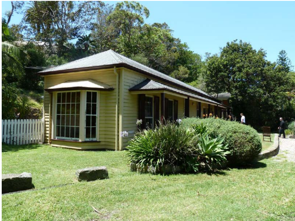
Figure 13 – Looking east towards Constables Cottages
