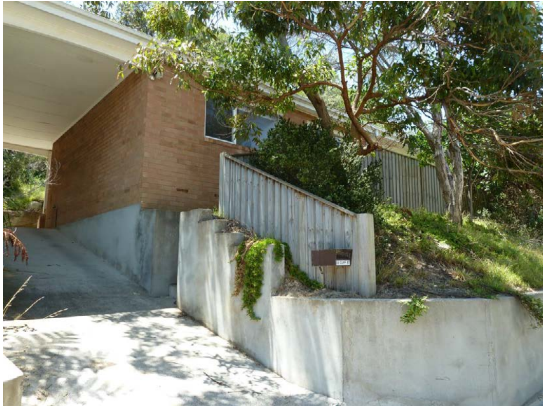
Figure 15 – 33 Cliff Street, as viewed from Cliff Street
