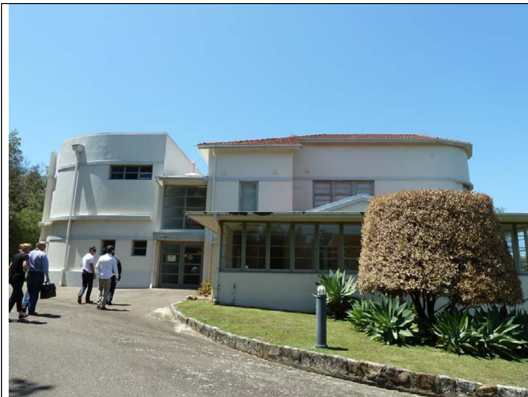
Figure 8 – The entry to the Officers Mess (western side)
