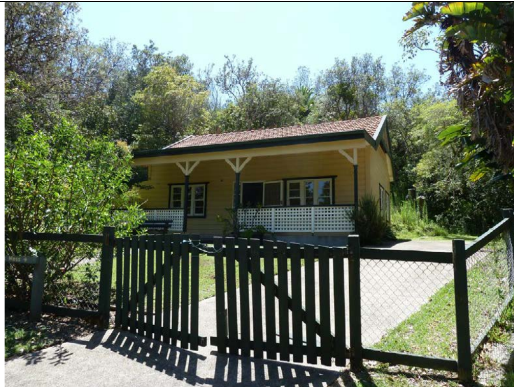
Figure 12 – Gap Bluff Cottage
