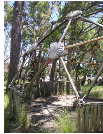
Picture 14 – South elevation
