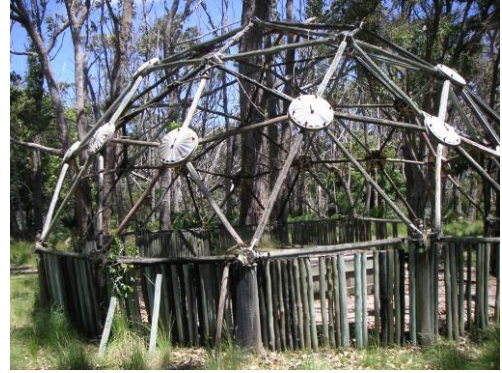
Picture 12 – General view of construction
