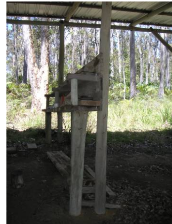
Picture 30 – Detail of bench under shed awning
