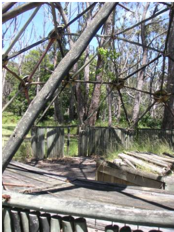
Picture 13 – Detail of base and internal area
