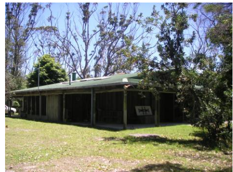
Picture 22 – South eastern corner of house
