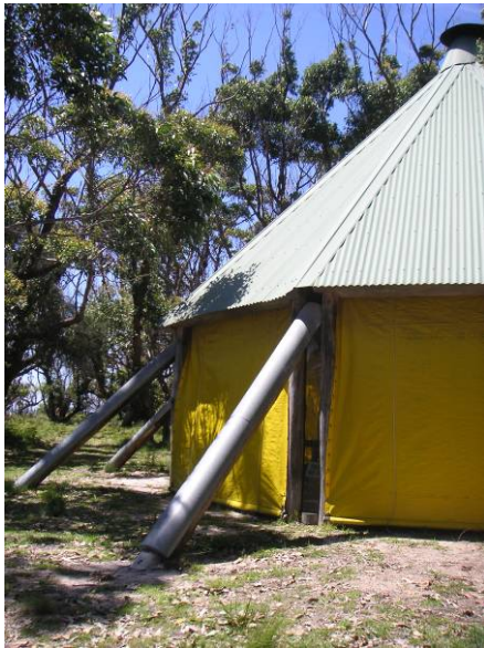
Picture 7 – External view
