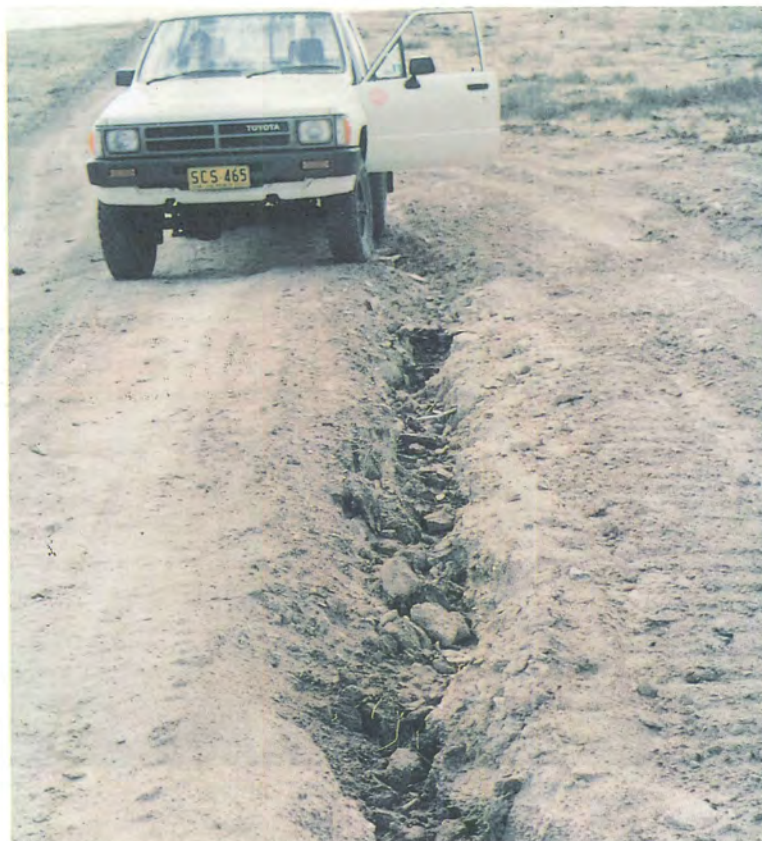
Plate 16: Rill erosion down formed access road. Also a common problem along poorly located and designed fire trails.
