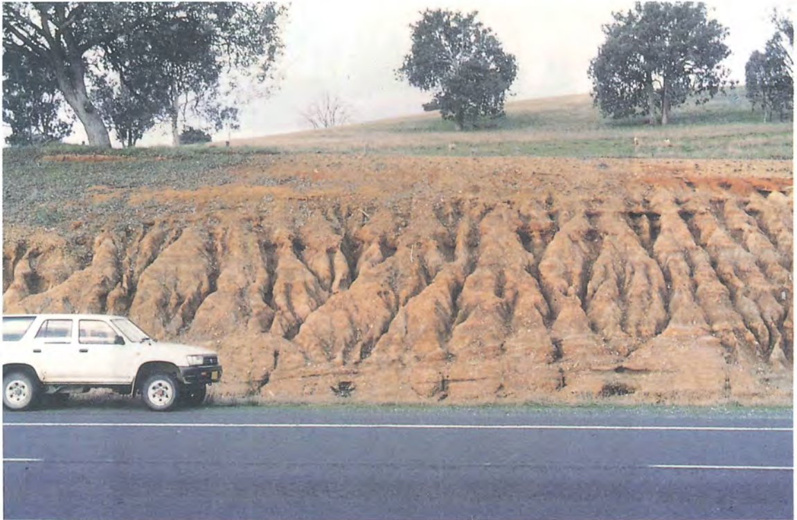
Plate 13: Rill erosion on a steep bare batter exacerbated by saline seepage. Photo Hume Highway. Mullengandra Creek catchment.
