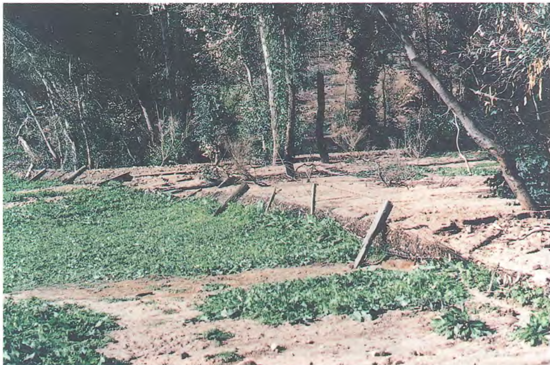
Plate 6: Sediment deposition resulting from severe sheet erosion caused by rains several months after wildfire. Photo Talmalmo area.
