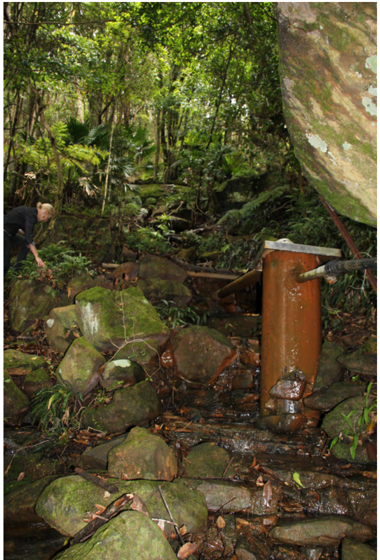
Figure 6.84 H1: Scout Camp Water Supply weir and primary filter
