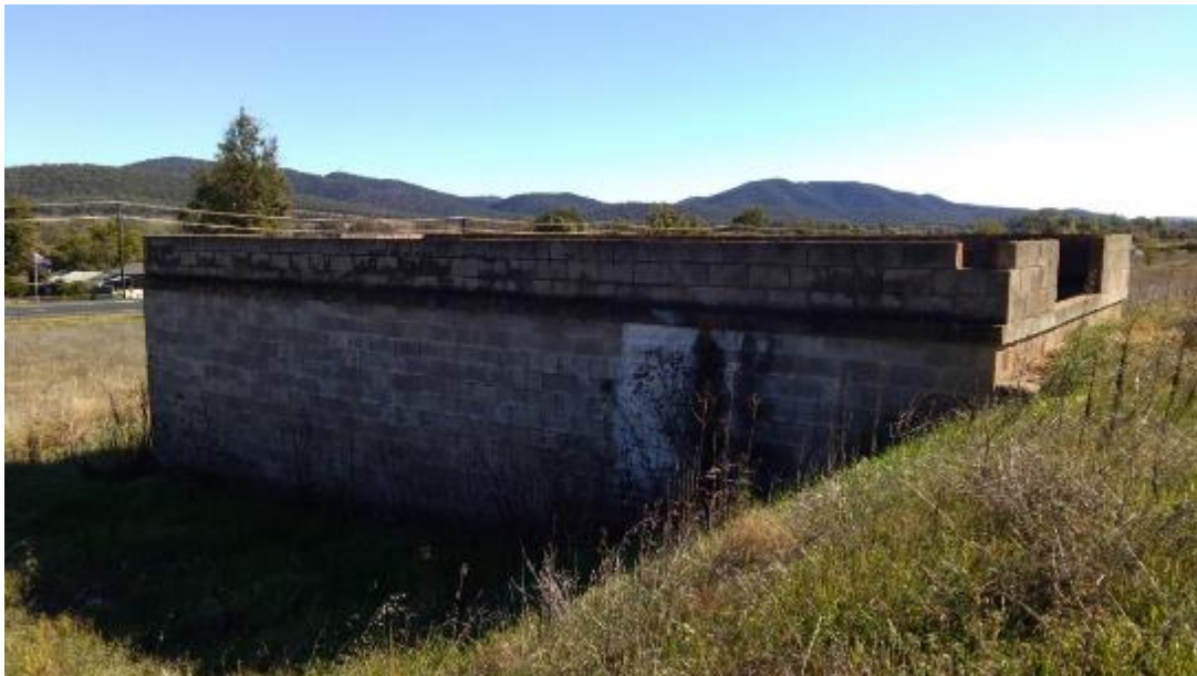
Photo 7 Besser block shed and loading ramp on Maynggu Ganai. M Billington/NPWS
