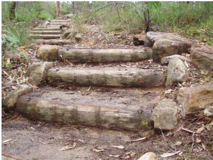
Example of half round TP timber steps (Edge rocks seen here are not necessary on most of the Coast Track steps)
