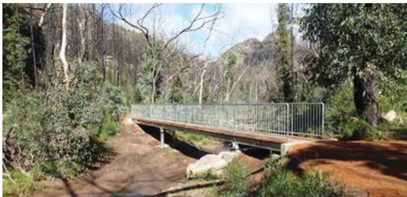
Steel frame and timber deck bridge at Warrumbungle NP
