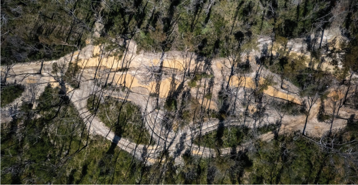
Existing site: Lost City access trail 4WD degradation and erosion.
