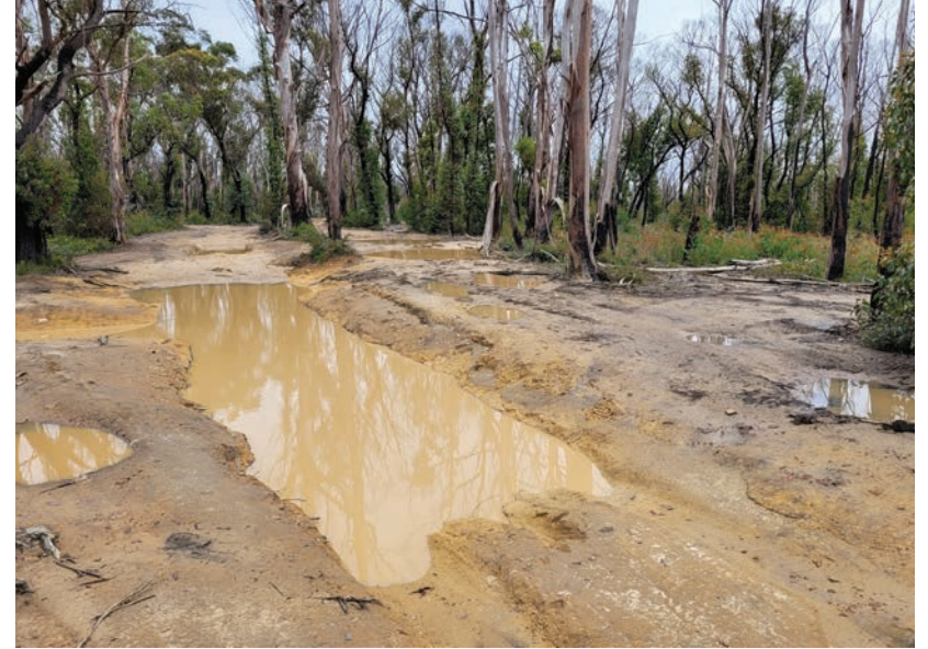
Existing site: Lost City access trail 4WD degradation and erosion.
