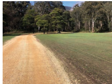
Crushed rock road
