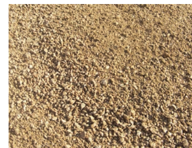
Stabilised gravel pavement
