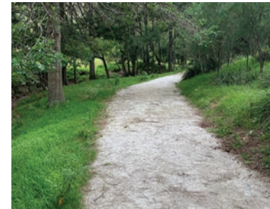
Crushed rock formed track
