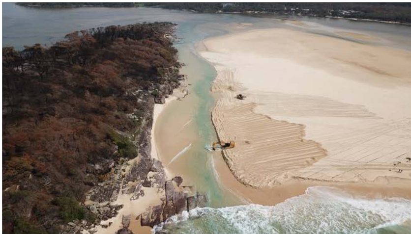
c) Excavation of the entrance channel 12 th Feb 2020
