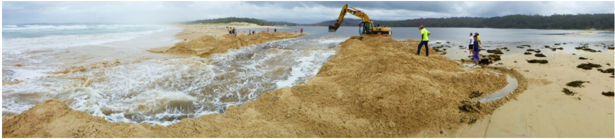
Photo 2 Mechanical opening of Lake Conjola on 10 February 2020 Photo: D Wiecek/DPIE.
