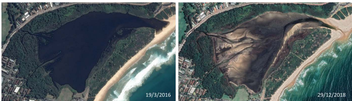
Figure 32 Complete drainage of Dee Why Lagoon following entrance breakout
