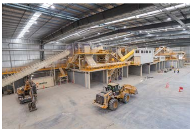
Top: The Boral Berrima cement works Above: The Cleanaway-ResourceCo facility in Wetherill Park, Sydney
