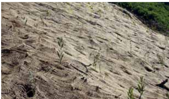
Hessian staked into the ground can help minimise water erosion
