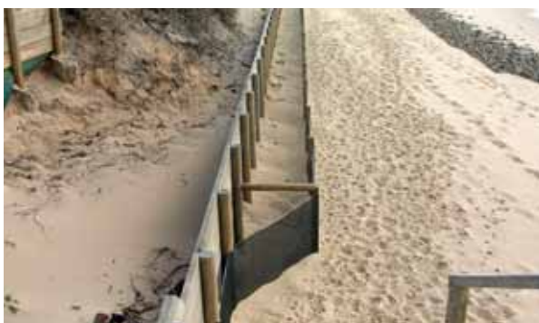
Timber and shade cloth fences can reduce wind erosion
