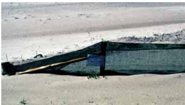
Shade cloth fence tapered at the end to minimise sand build up
