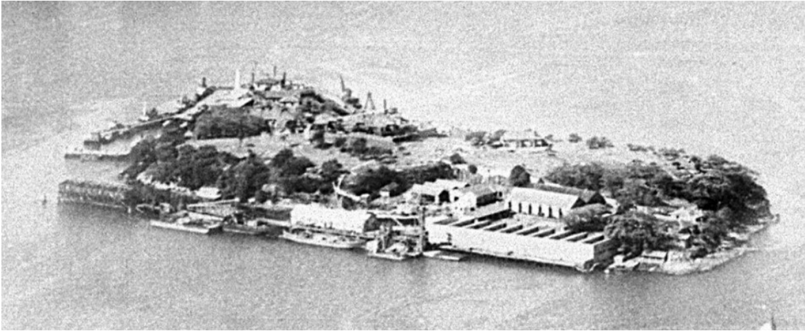
Figure 21: Goat Island, looking south over the shipyard towards East Balmain prior to the relocation of the crane in 1962 (Former MSB Archives MSBL1425).
