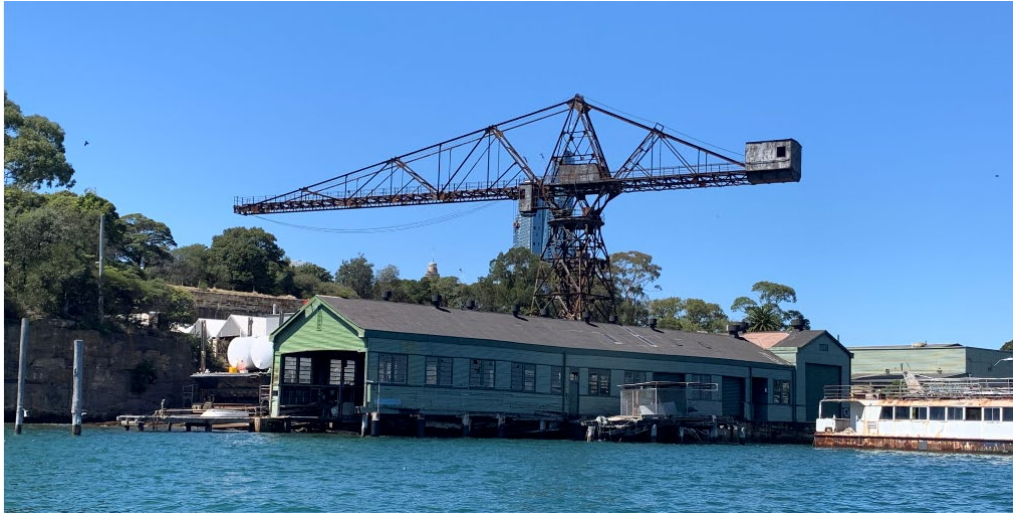
Figure 308: The Tower Crane over the Shipyard and Magazine precincts (R Newton/NPWS)
