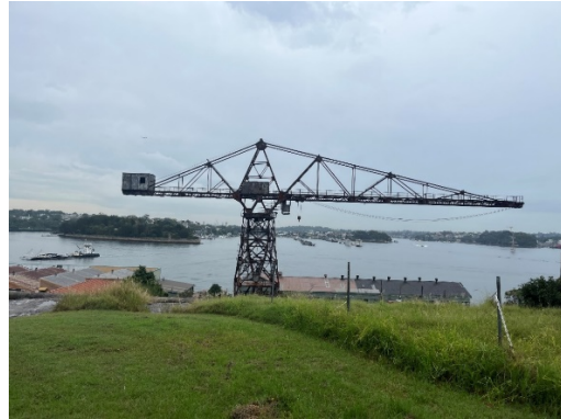
Figure 10: View west from the ridge of Goat Island across the Tower Crane to Birchgrove and Greenwich (Source: Artefact February 2024)
