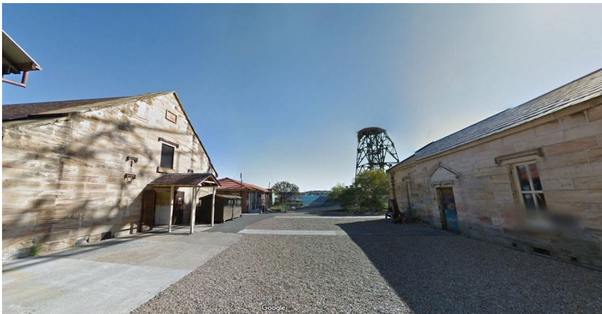
Figure 52: The westward view from the Powder Magazine precinct partially recaptures the qualities of the skyline before the crane was erected.
