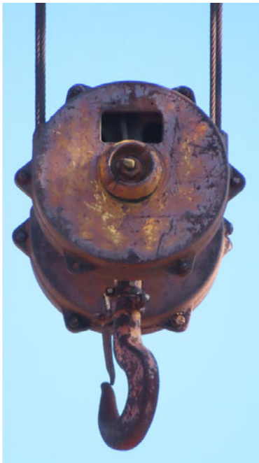
Figure 249: The crane hook (R Newton/NPWS, 2024)
