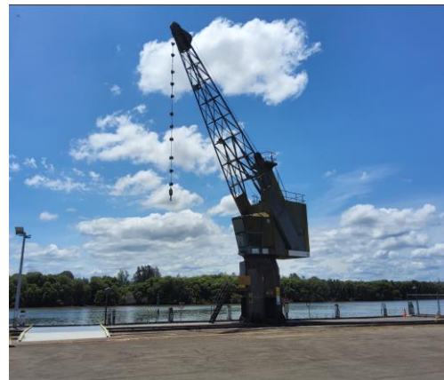
Figure 207: The Newington Armory Eastern Crane (Ed Beebe/NPWS)
