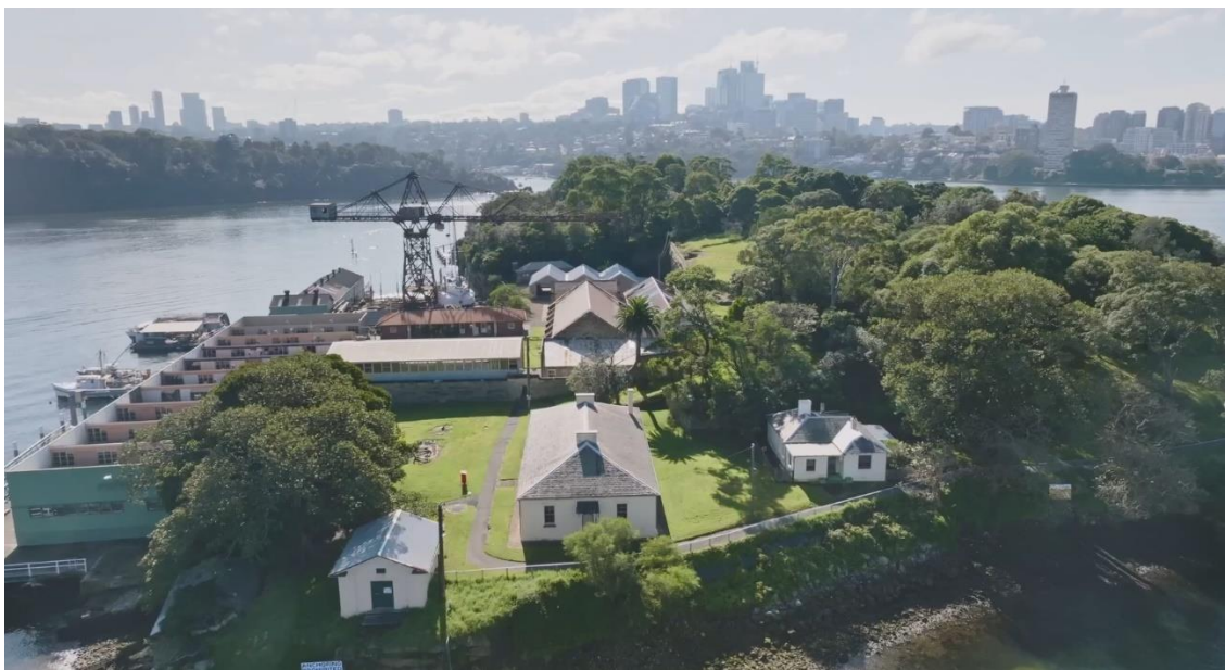
Figure 37 The Tower Crane over-sailing the Powder magazine Cooperage (NPWS 2022)
