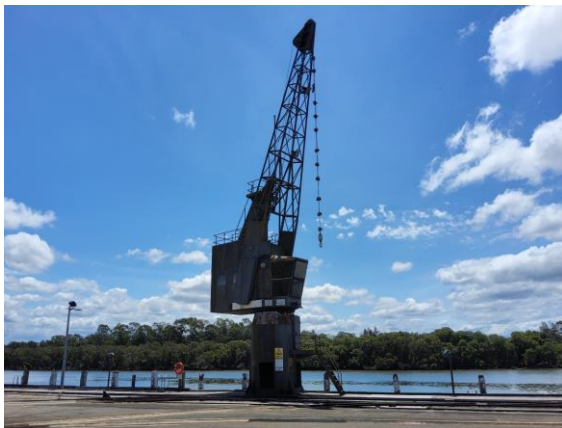
Figure 196: The Newington Armory Western Crane (Ed Beebe/NPWS)
