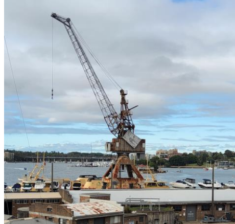
Figure 106: Southerland Wharf Electric Portal Travelling Jib Crane, Crane Number C277 (NPWS/Ed Beebe Nov 23)
