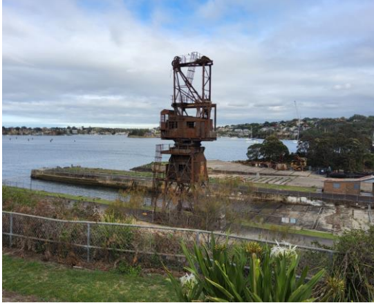
Figure 95: Northern Slipway Travelling Crane, Crane Number C300, with jib removed since 2019 for safety (Ed Beebe/NPWS)
