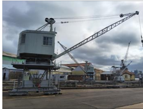
Figure 128: The southern of the two Electric Travelling Jib Cranes, AFD Crane 2, Crane Number C227 (Ed Beebe/NPWS)
