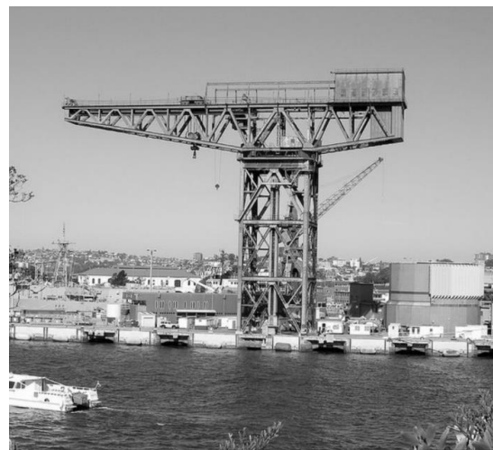
Figure 10: The Garden Island 250T cantilever crane
