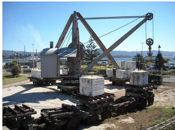
Figure 163: More recently, the crane in April 2013 (Wollongong Council)
