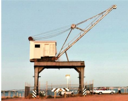
Figure 7: Arrol designed Bunbury Jetty Crane 1911 (inherit.stateheritage.wa.gov.au)
