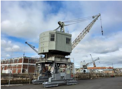
Figure 117: The northern of the two Electric Travelling Jib Cranes, AFD Crane 1, Crane Number C226 (NPWS/Ed Beebe)
