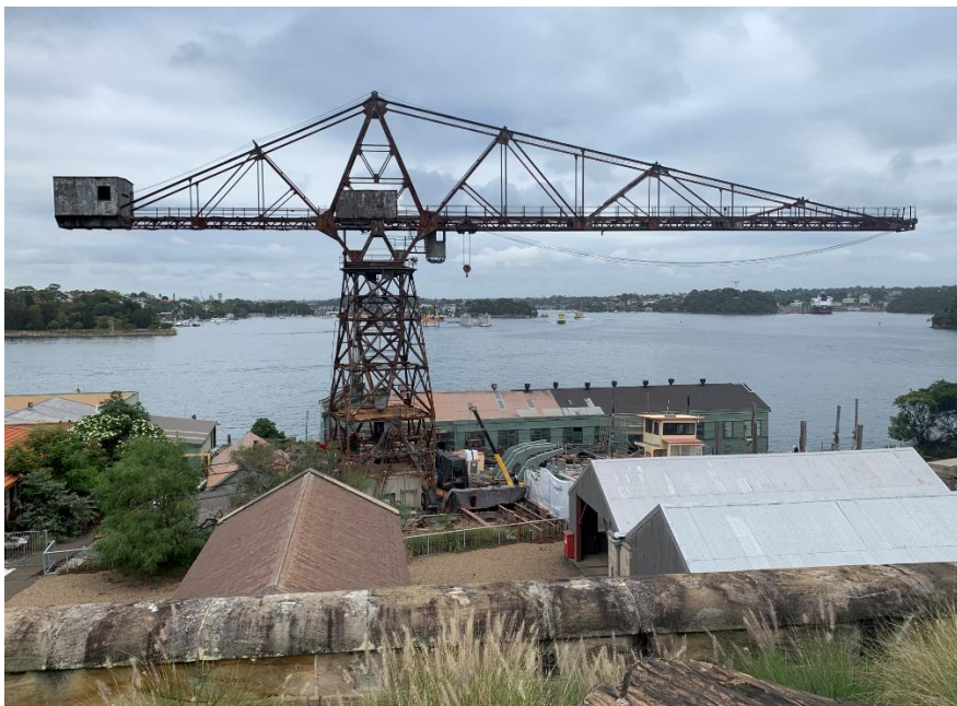
Figure 6: The Magazine Precinct viewed from the island's western ridge (R Newton/NPWS)
