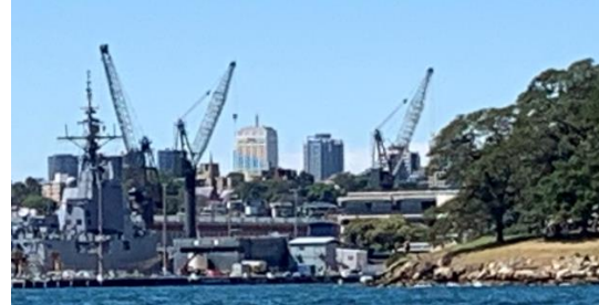
Figure 12: Three of the four large cranes operating at Garden Island (R Newton/NPWS).
