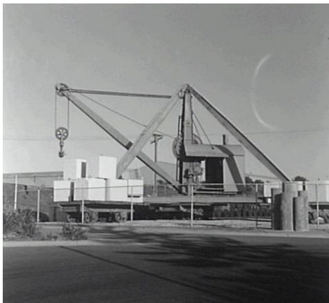
Figure 152: Mobile Block Setting Steam Crane (Wollongong Council)
