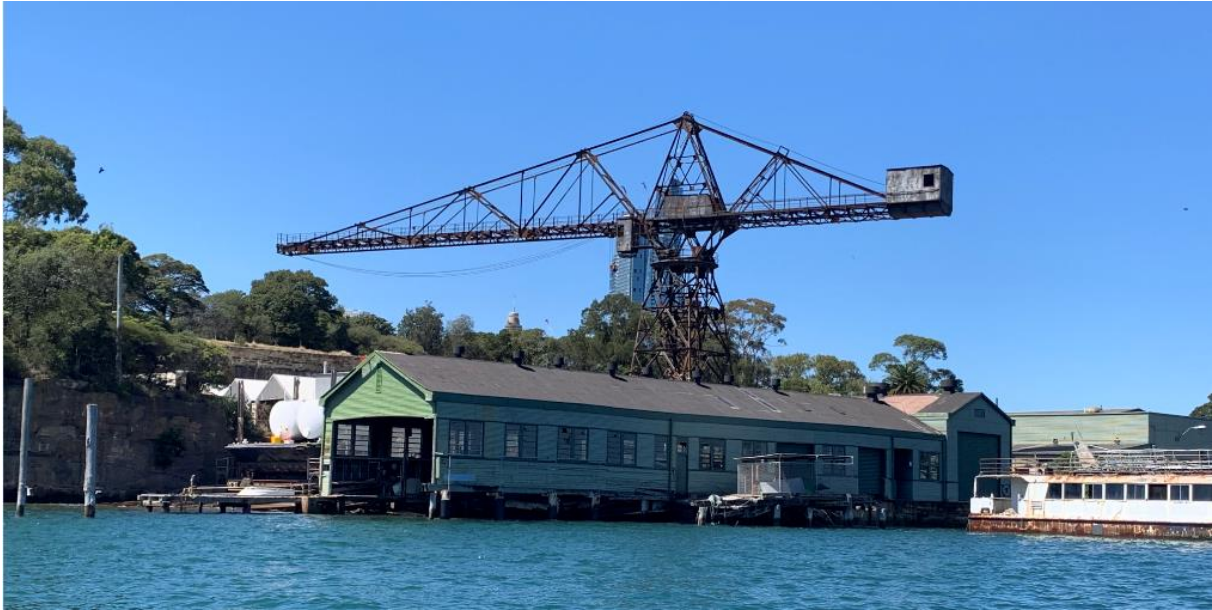
Figure 5: The Tower Crane over the Shipyard and Magazine precincts (R Newton/NPWS)
