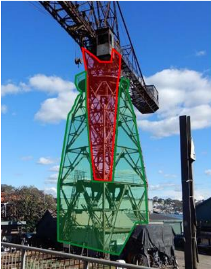
Figure 2 - View on the outer tower (green shape) and the inner tower and slew mechanism (red shape)
