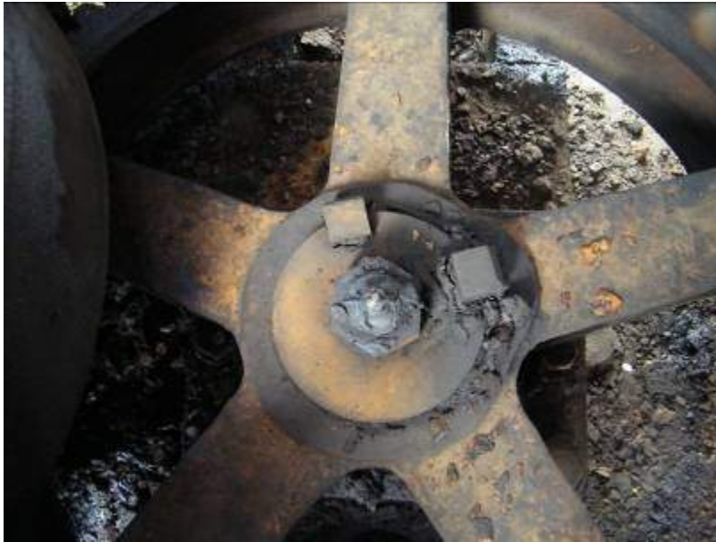
Figure 8 Worn Keyway on main slewing gear
