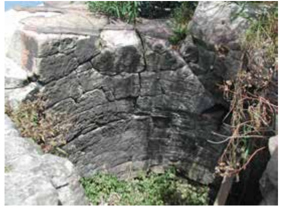
Detail, lime kiln
