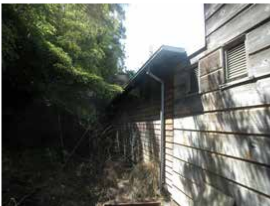
Timber store north elevation
