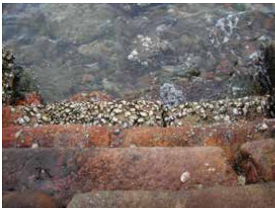
Detail, stone jetty
