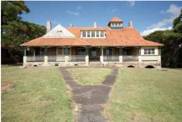
East elevation, Harbour Master's residence
