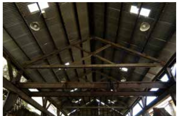
Scow Shed interior, detail of roof truss system
