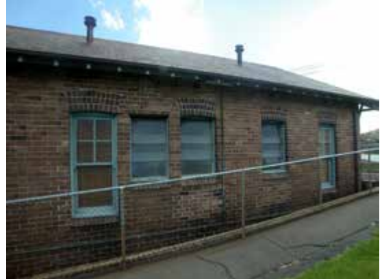
Fire Brigade Barracks, detail of western end of north elevation, showing window alterations
