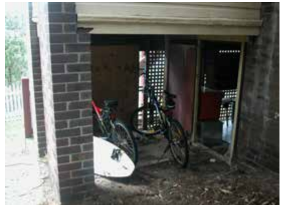
Detail, undercroft beneath front verandah
