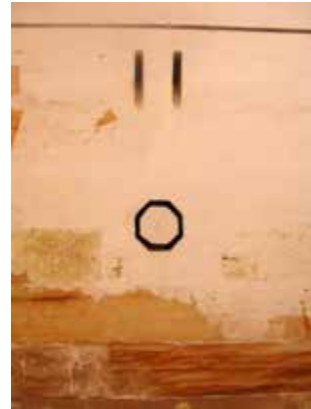
Baffled vent from interior of Queen's Magazine. Note damage from damp penetration below.
