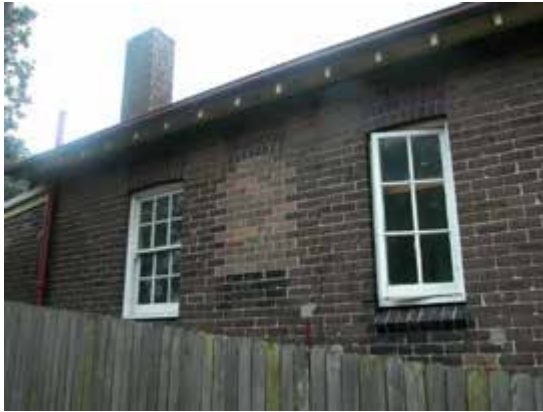
Detail, south elevation, Residential Cottage No. 4, showing brick infill of former window opening
