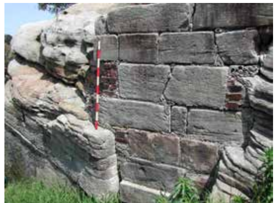
Detail, lime kiln
