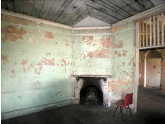
Interior, Water Police Station. Note early 20th century alterations: mantelpiece and screen, wider doorway opening
