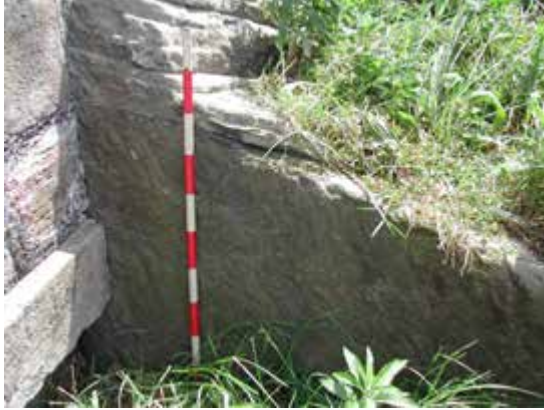
Detail, lime kiln
