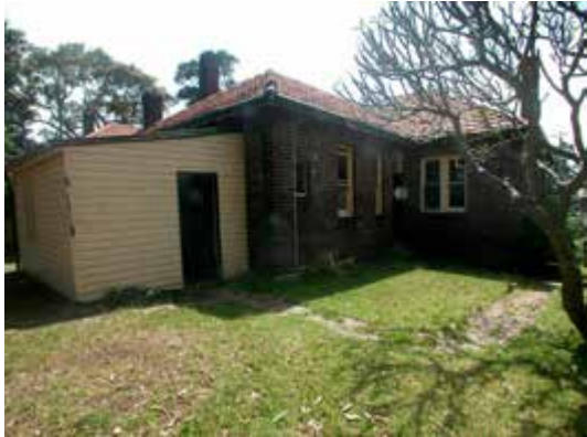
Rear of south elevation Residential Cottage No. 2
