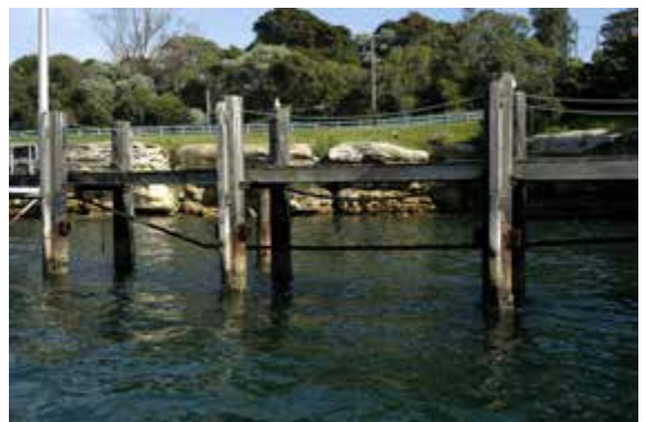
Detail, Wharf mooring floating plant
