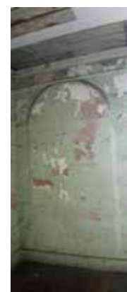
Interior, blocked up doorway to west elevation
