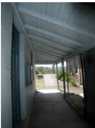
View along north verandah of Cottage
