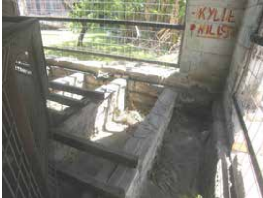
Exposed floor structure in eastern bay
