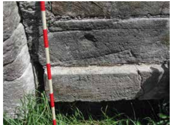
Detail, lime kiln
