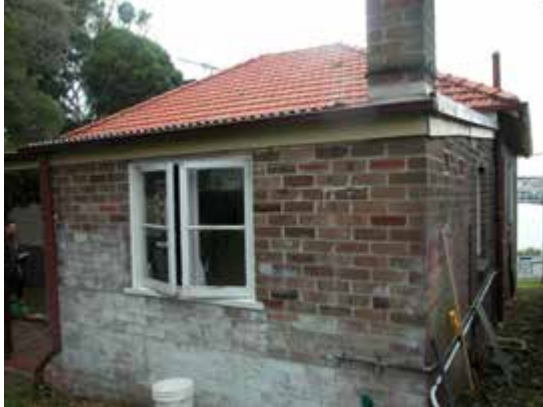
Detail, brick rear laundry extension
