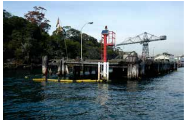
Coal Bunker platform from the north
