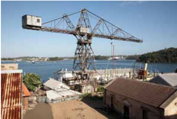
Hammerhead crane from the east
