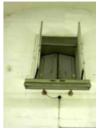
Double timber shutters to north end of Queen's Magazine, taken from interior
