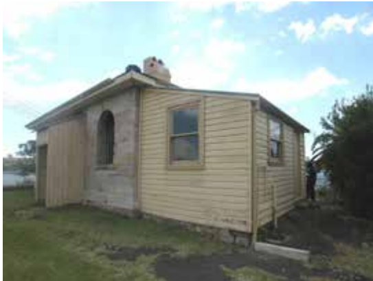
Water Police Station west elevation to right, part south elevation to left, with later weatherboard addition.
