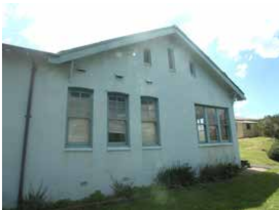
Fire Brigade Barracks, detail of east elevation. Set of three windows at right are clearly a later addition.
