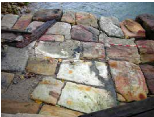
Detail, stone jetty
