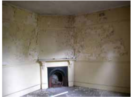
Living room corner fireplace, Residential Cottage No. 3
