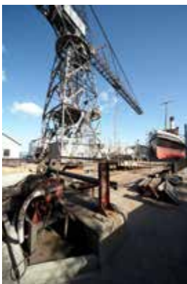
Base of Hammerhead crane
