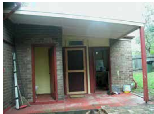
Detail, north elevation of rear brick wing
