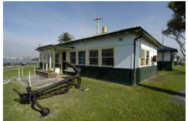
Dredge office, east and north elevations
