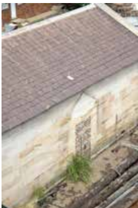
Cooperage north elevation showing bricked up entry door which once connected to a covered way leading to the Colonial Magazine.
