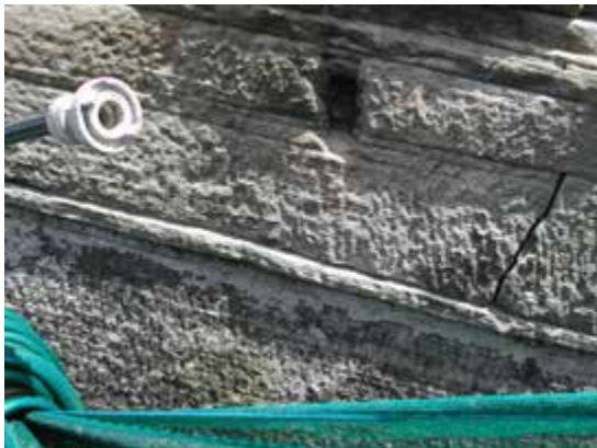
Detail, lime kiln
