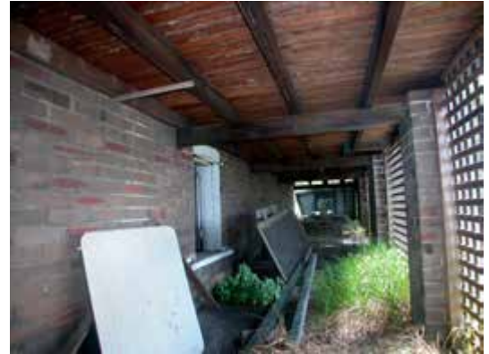
Detail, undercroft area beneath front verandah
