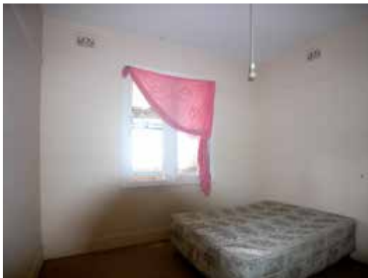
Typical interior, front bedroom. Note no cornices.
