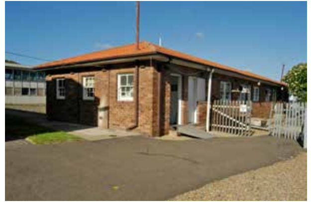
1948 Amenities building, east and north elevations
