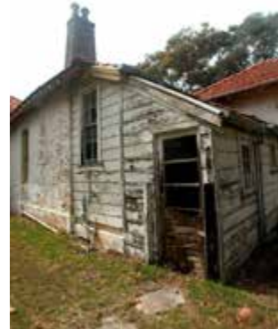
Detail, weatherboard addition
