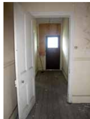
View towards front door, Residential Cottage No. 3. Note modern flush front door, plywood over fanlights, sidelight
