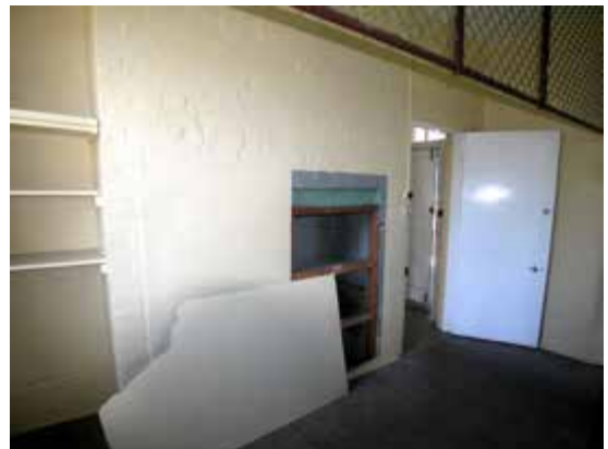
Southern room of cottage, showing later door, original hearth with later shelving, part of clothing racks, part of entry vestibule and main entry door visible through the door
