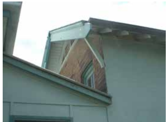
Detail, Fire Brigade Barracks, junction of verandah roof of Cottage 46a on left with gable end to Fire Brigade Barracks at right
