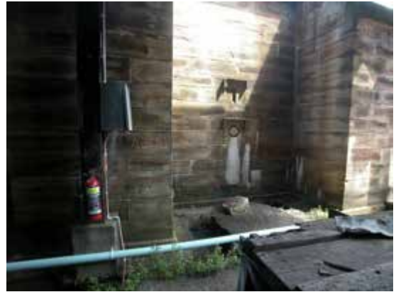
Detail, west side of Scow shed interior, showing floor of Scow shed excavated away from the east wall of the Queen's Magazine
