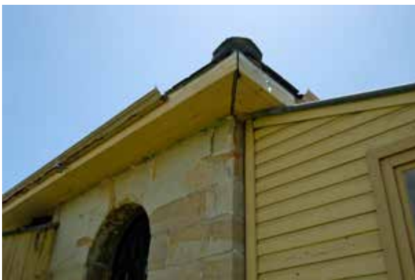
Water Police Station, detail of eaves
