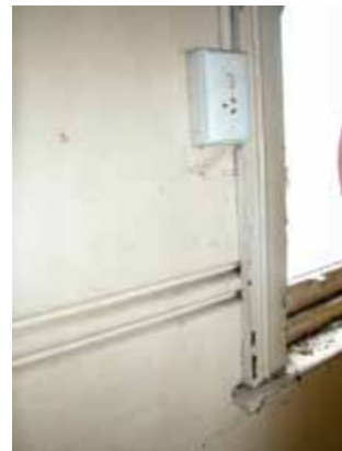
Chair rail moulding, Residential Cottage No 3
