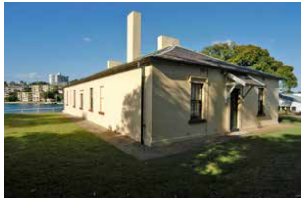
North and east elevations, Barracks
