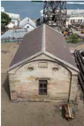
Cooperage from east, above
