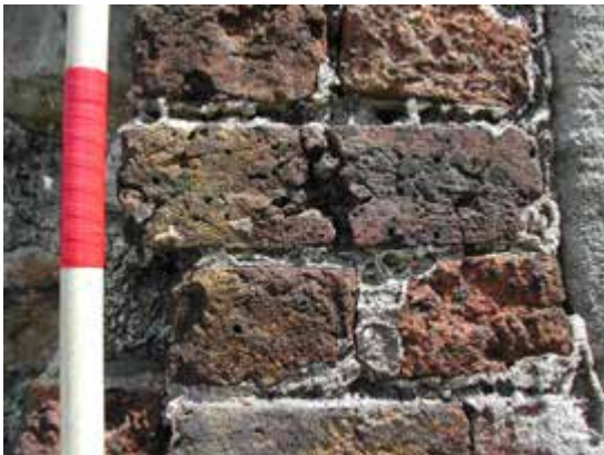
Detail, lime kiln
