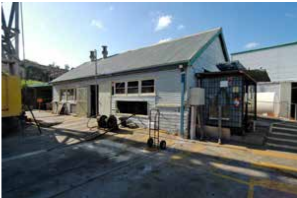
150 ton slipway winch house
