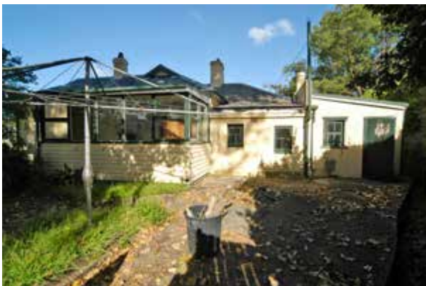
East elevation, kitchen cottage
