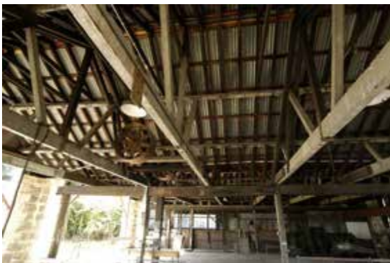
Colonial Magazine interior, roofing detail
