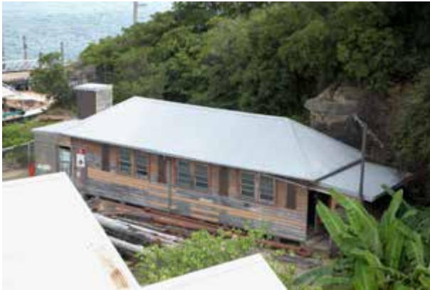
Timber store south elevation from above
