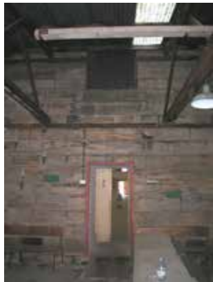
Doorway and door to southern elevation, from interior of southern addition to the Queen's Magazine. Note copper screen to southern window opening intact above the doorway.
