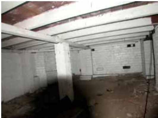
Detail, floor structure from undercroft
