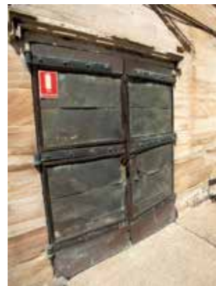
Copper-sheathed entry doors, north elevation, Queen's Magazine
