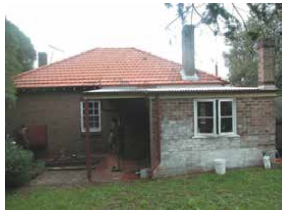
Rear (west) elevation, Residential Cottage No. 4, showing 3 chimneys to roof, and brick rear laundry extension
