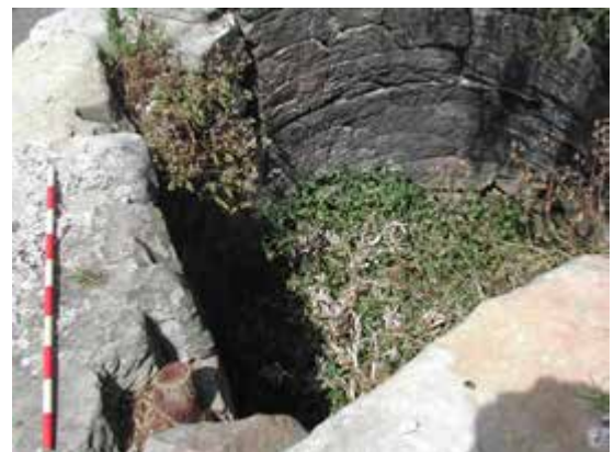
Detail, lime kiln
