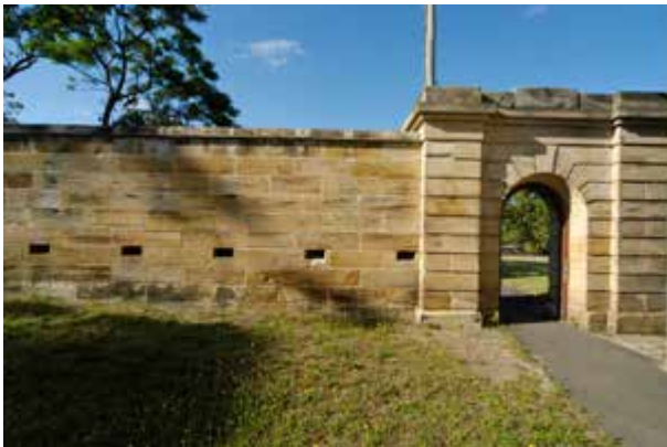
Fortified wall and entry from northern side
