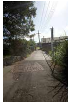
Looking across the bridge over Barney's Cut
