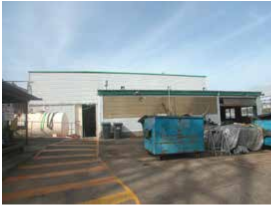
North elevation, with addition in foreground
