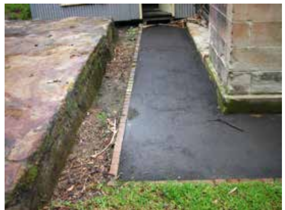
Detail of quarrying evidence near Stores Building (20)
