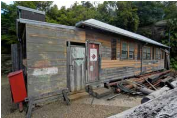
Timber store south elevation from west
