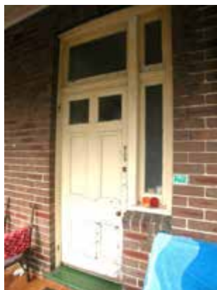
Detail of front door, fanlights, sidelight
