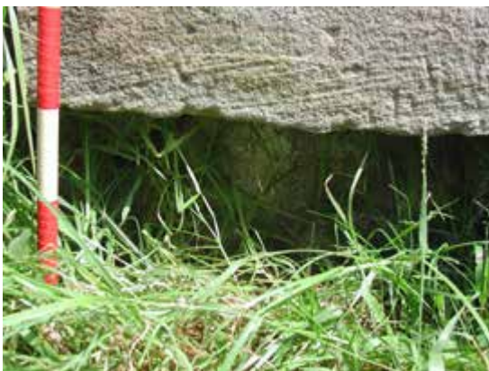
Detail, lime kiln
