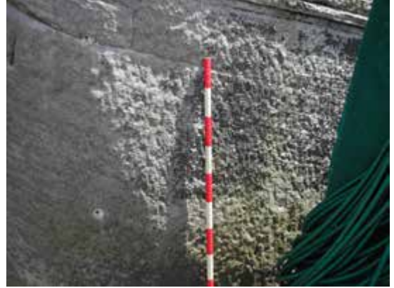
Detail, lime kiln
