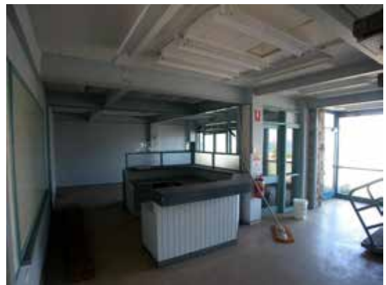
Interior, first floor, Port Emergency Services Building
