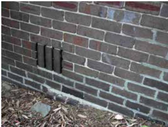
Detail, vent to footing
