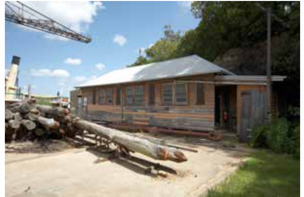
Timber store south elevation
