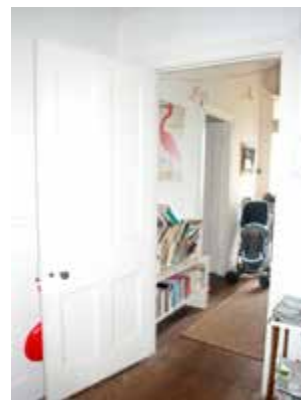
Typical internal 4-panel timber door
