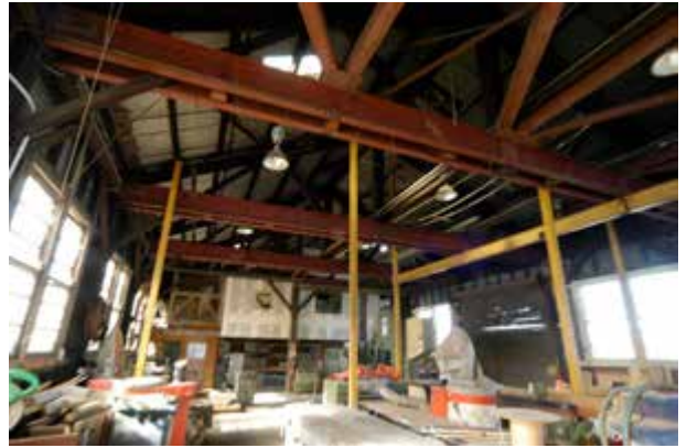
Interior, Repair Workshop and Repair Workshop extension
