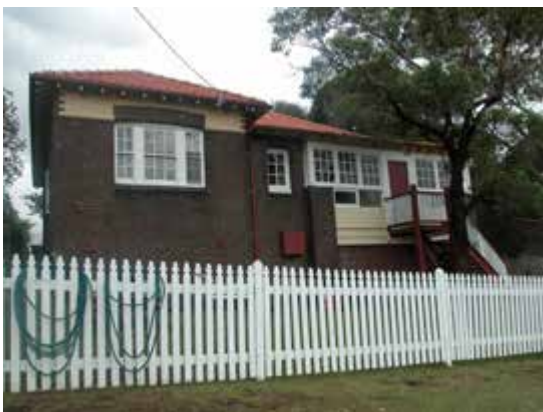
Detail front (east) elevation, Residential Cottage No. 4
