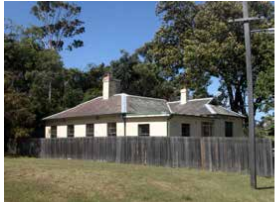
West and south elevations, Kitchen Cottage.
