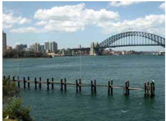
Southern end of Wharf mooring floating plant
