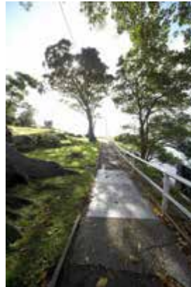
Magazine walk near Kitchen Cottage (26) looking northeast
