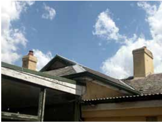
Roof and chimney detail, Kitchen cottage
