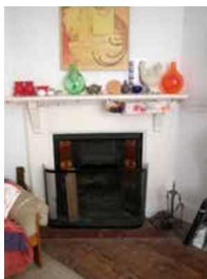
Fireplace to living room
