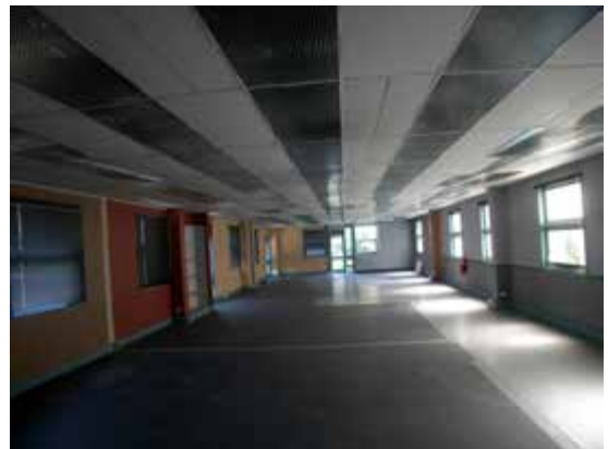
Interior, first floor, Port Emergency Services Building
