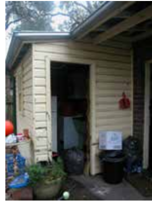
Southern elevation of weatherboard laundry
