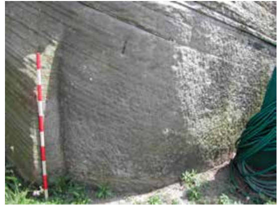
Detail, Lime Kiln
