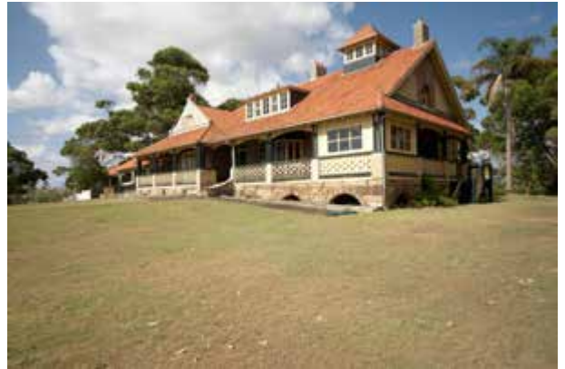
East and north elevations, Harbour Master's Residence
