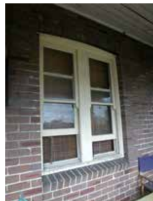
Detail of front windows to east elevation
