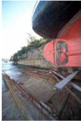
500 ton slipway looking north
