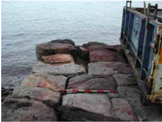
Detail, stone jetty
