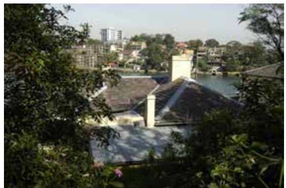
Roof detail, Kitchen cottage
