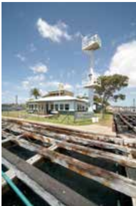
Dredge office from east
