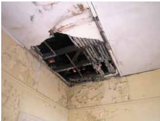
Damage to plaster ceiling of living room, showing exposed timber battens, Residential Cottage No. 3
