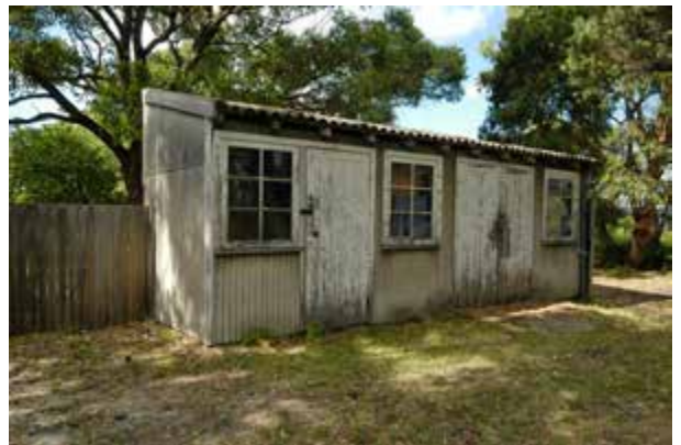
Rear shed, Harbour Master's Residence
