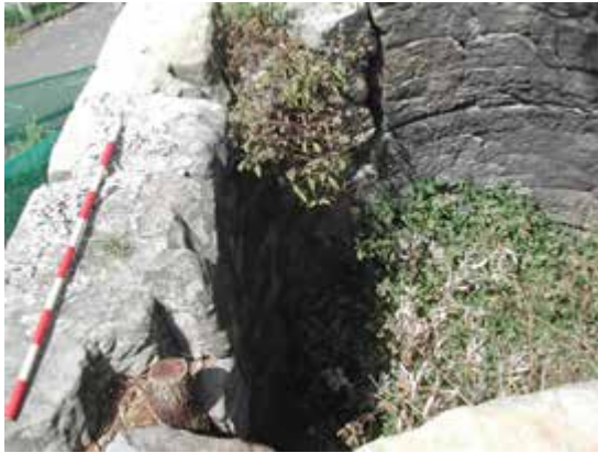
Detail, lime kiln
