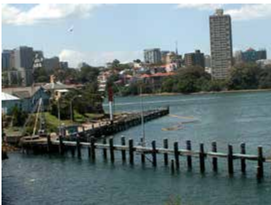
Northern end of Wharf mooring floating plant
