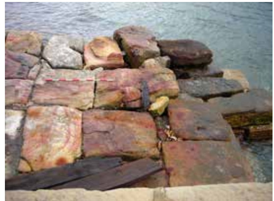
Detail, stone jetty
