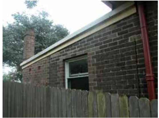
Detail, rear (west end) of south elevation, showing alterations to brickwork indicating insertion of new window, and brick rear laundry extension with chimney
