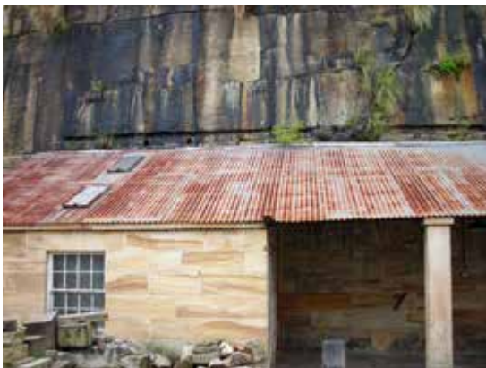
Magazine Quarry face behind Stores Building (20)
