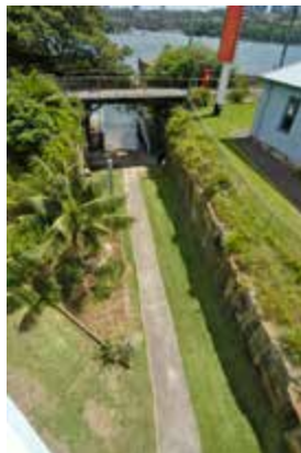
Bridge over Barney's Cut
