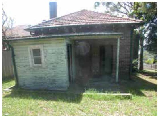
Rear (west) elevation, Residential Cottage No. 3
