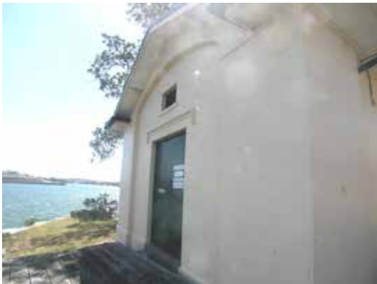
Transformer house, south elevation, facing the harbour
