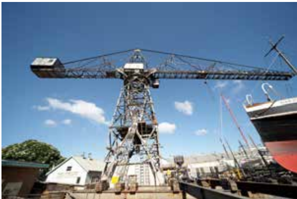
Close view of hammerhead crane
