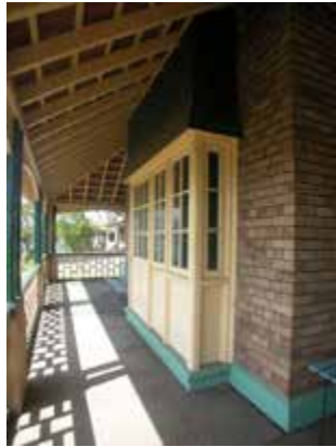
View down front verandah from north
