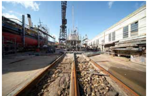
150 ton slipway. Repair Workshop to right.
