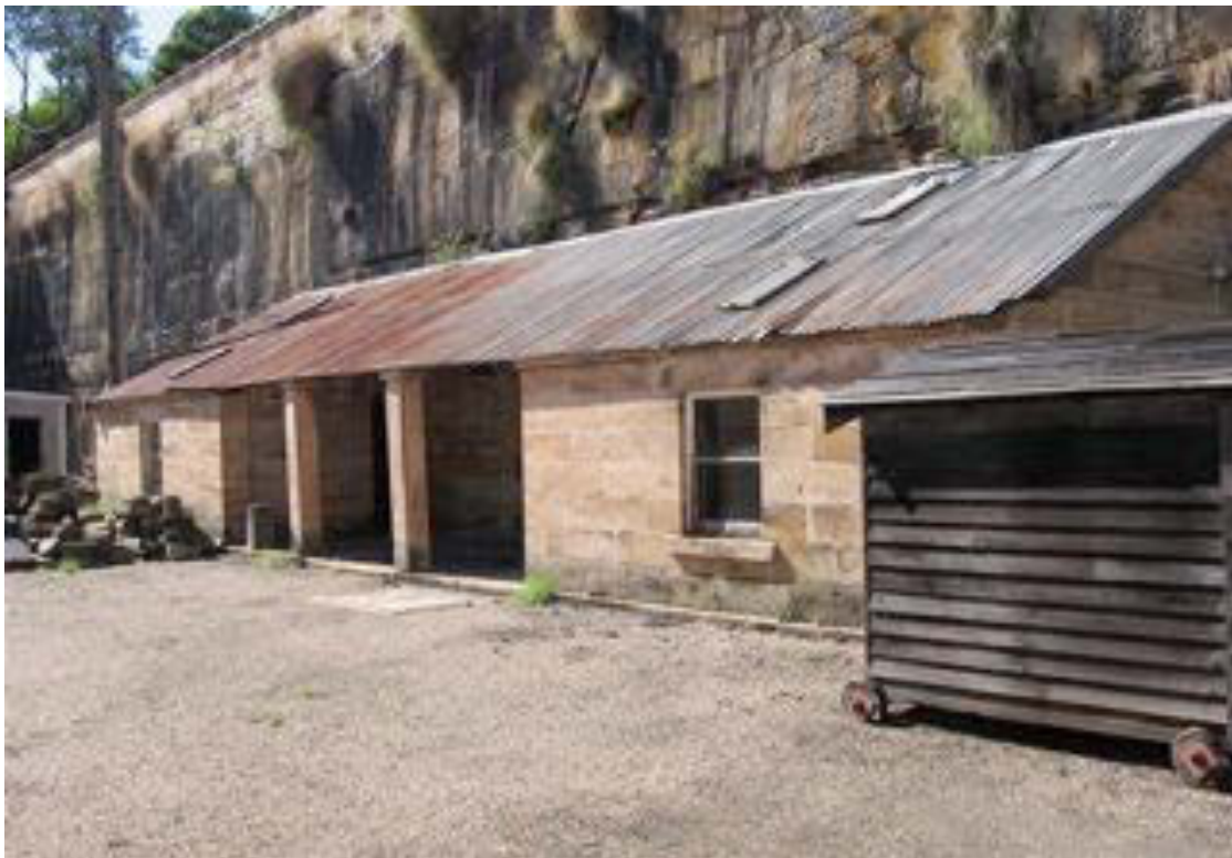
Figure 35: Stone shed (cooperage) built against the quarry wall in 1839 – view NE (2007)
