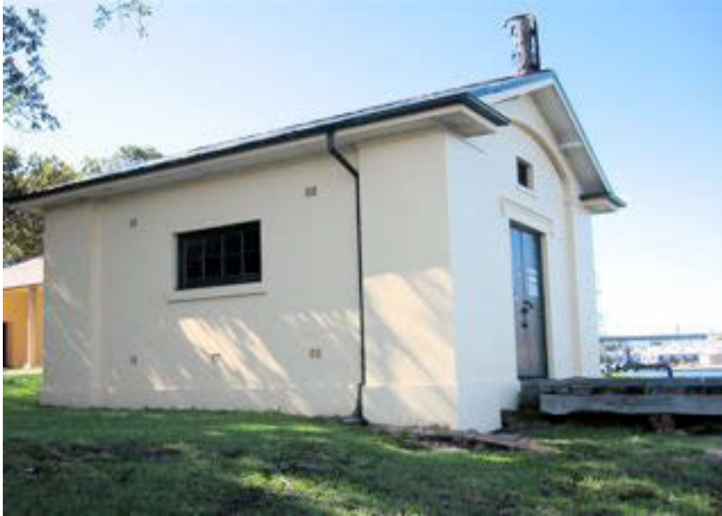
Figure 91: Goat Island Transformer House – view NE (2007)
