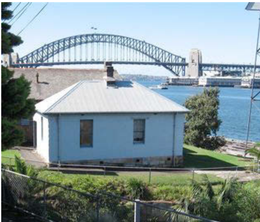
Figure 51: Labourer's Cottage 1865 - view ESE (2007)
