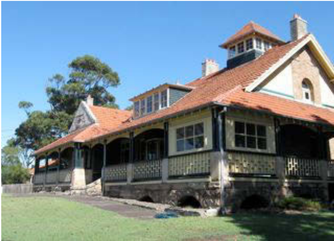
Figure 72: Harbour Masters Residence c.1902/03 – view SSW (2007)
