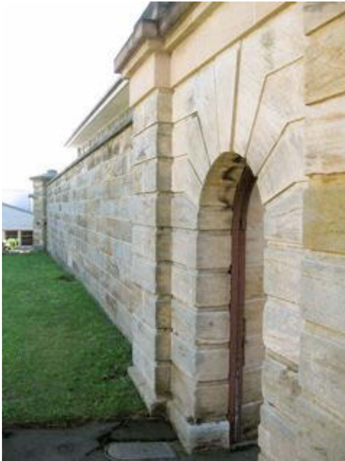
Figure 36: Perimeter wall around the magazine precinct - view WNW (2007)
