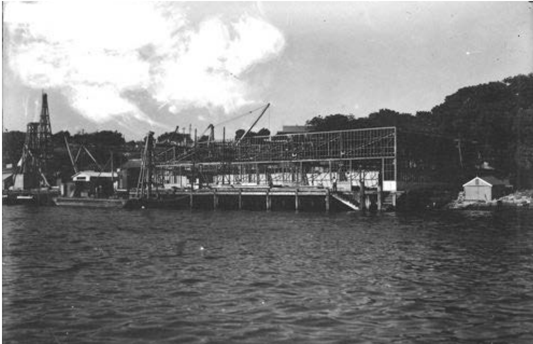
Figure 94: Construction work in the Goat Island shipyard (n.d.)
