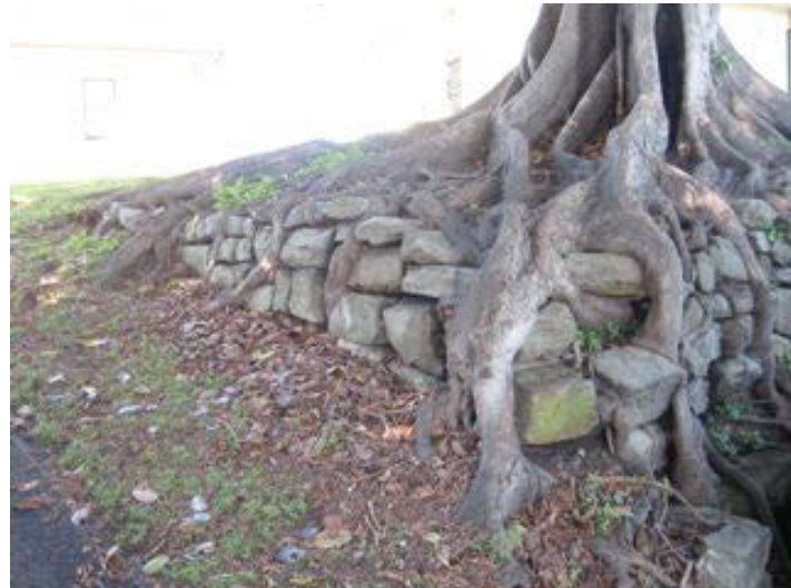
Figure 9: Port Jackson Fig roots Port Jackson fig roots morphing with an historic sandstone retaining wall near the barracks building on the southwestern tip of Goat Island.
