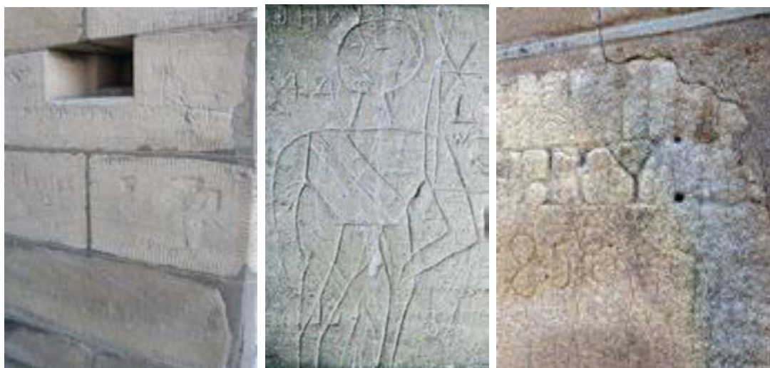
Figure 56: Garrison graffiti on the Magazine precinct sentry box and perimeter wall (2007)
