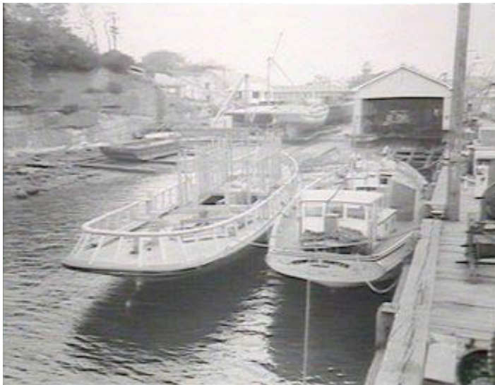
Figure 101: Construction of vessels: Goat Island (November 1952)
