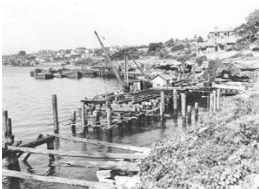
Figure 89: 'Wharf construction, Goat Island' (n.d.)
