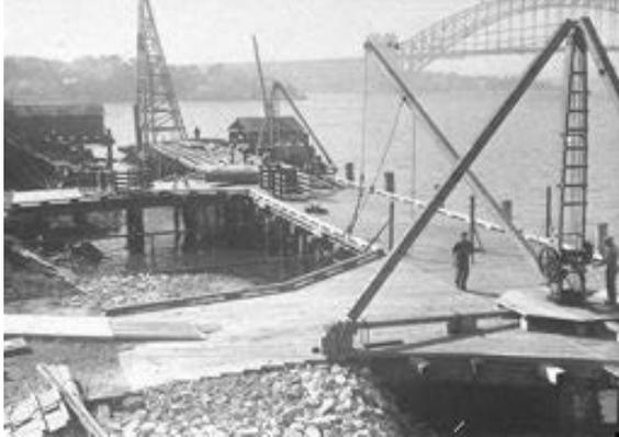
Figure 2.18 Reconstruction of the eastern wharf.
