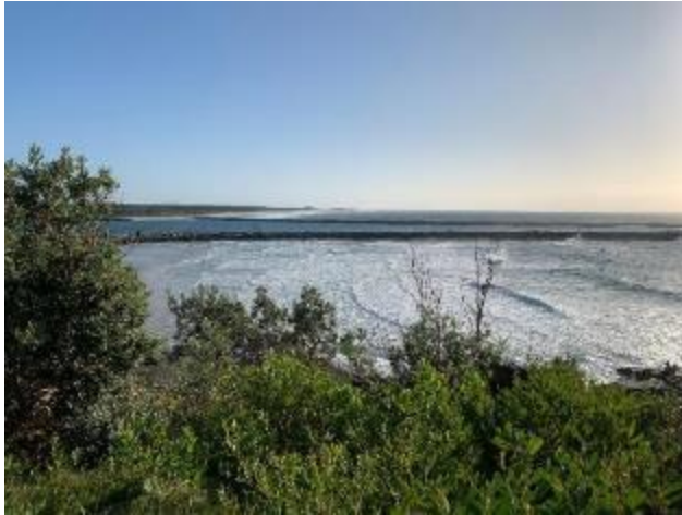
1 – Clarence River entrance breakwaters
