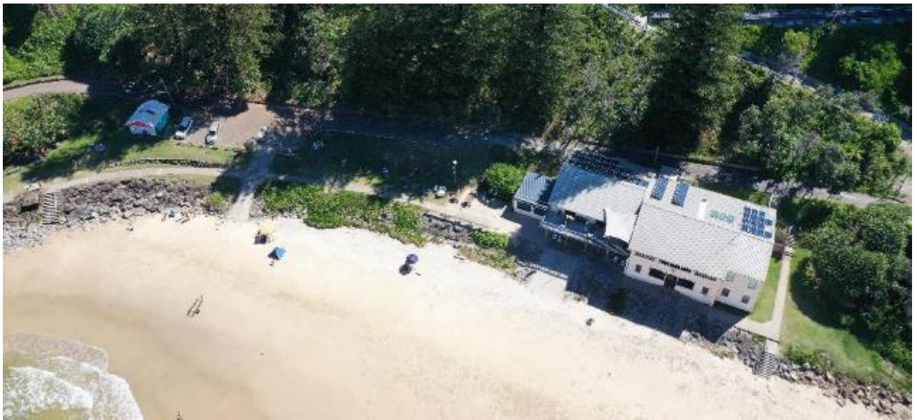
Plate 6: Yamba SLSC and Yamba Main Beach revetment wall (February 2022)
