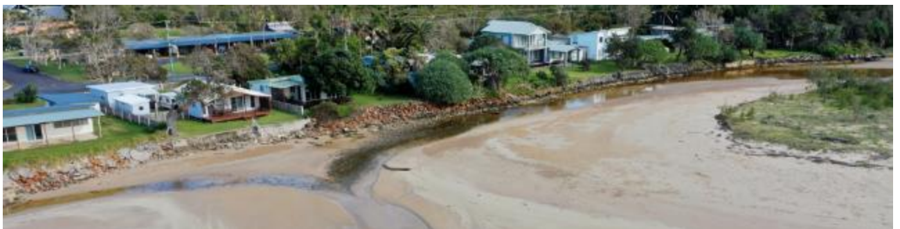
Plate 9: Informal protection works and private properties between the foreshore and Ocean Road
