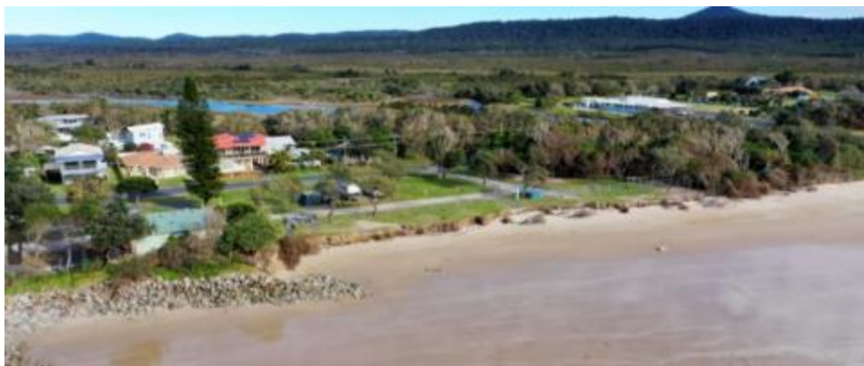
Plate 8: Erosion along northern end of Brooms Head Holiday Park (June 2022)
