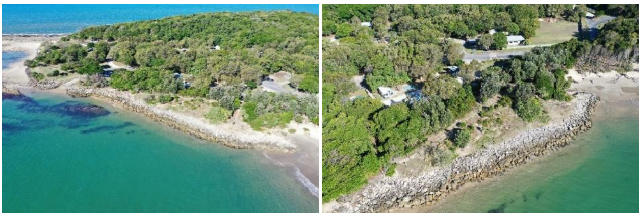
Plate 13: Woody Head campground seawall (Plate 13-L, Plate 13-R)
