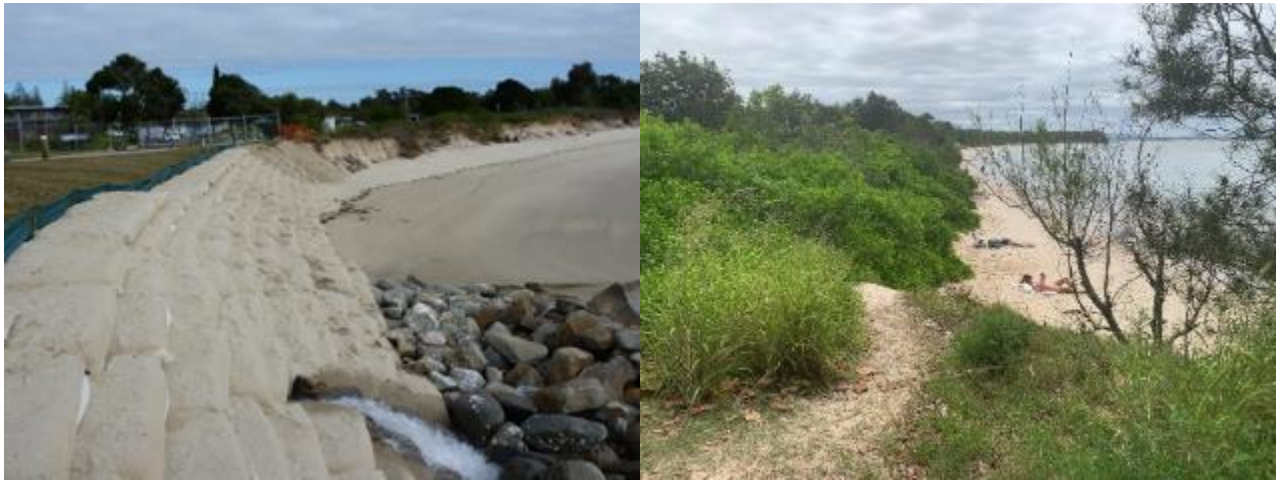
Plate 5: Left: geobags constructed at Whiting Beach (2012/13), right: vegetation has regrown with crest of the wall exposed by informal pedestrian access (January 2024)
