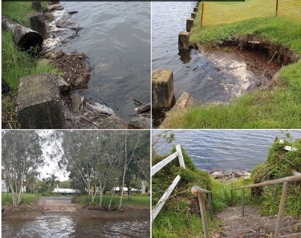
Figure 10 Damage to infrastructure at Mylestom Reserve foreshore.
