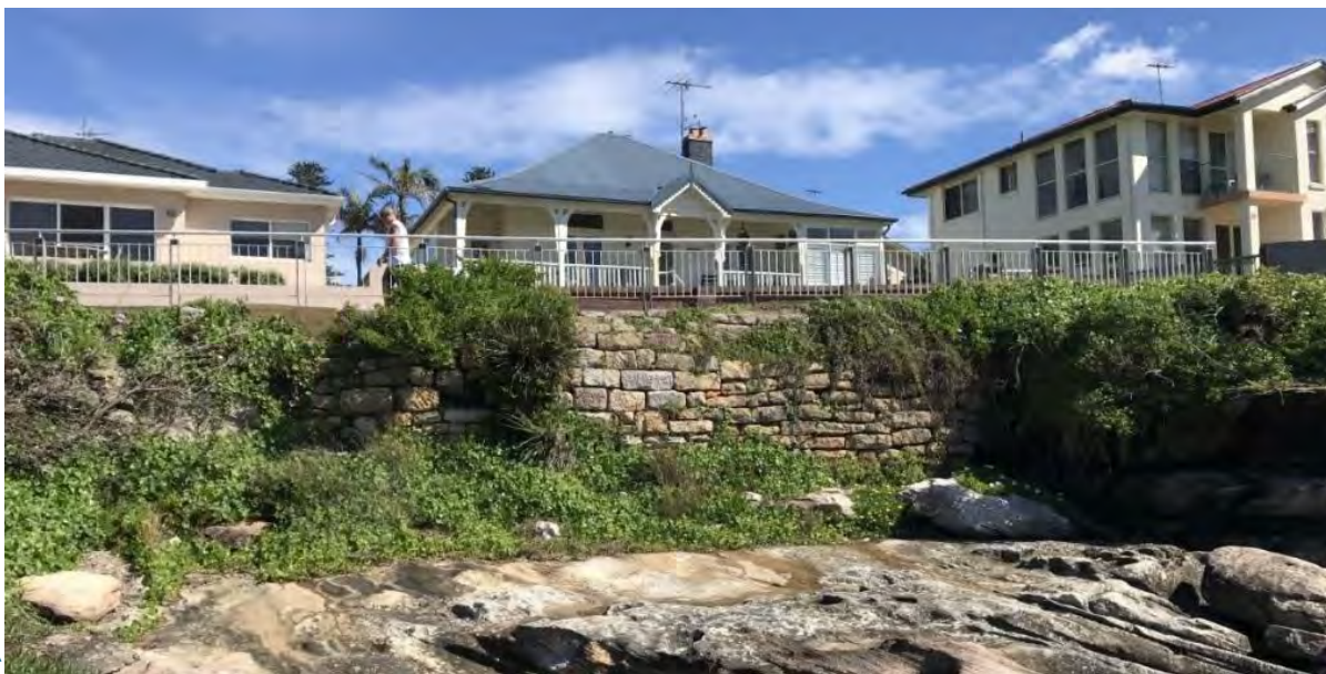
Figure 8-1: Loosely Stacked Sandstone Masonry Wall opposite No. 88 and 87 The Esplanade
