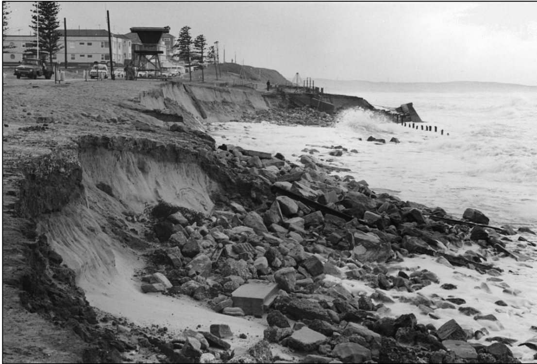
Figure 3-11: 1974 Storm Erosion at North Cronulla Beach
