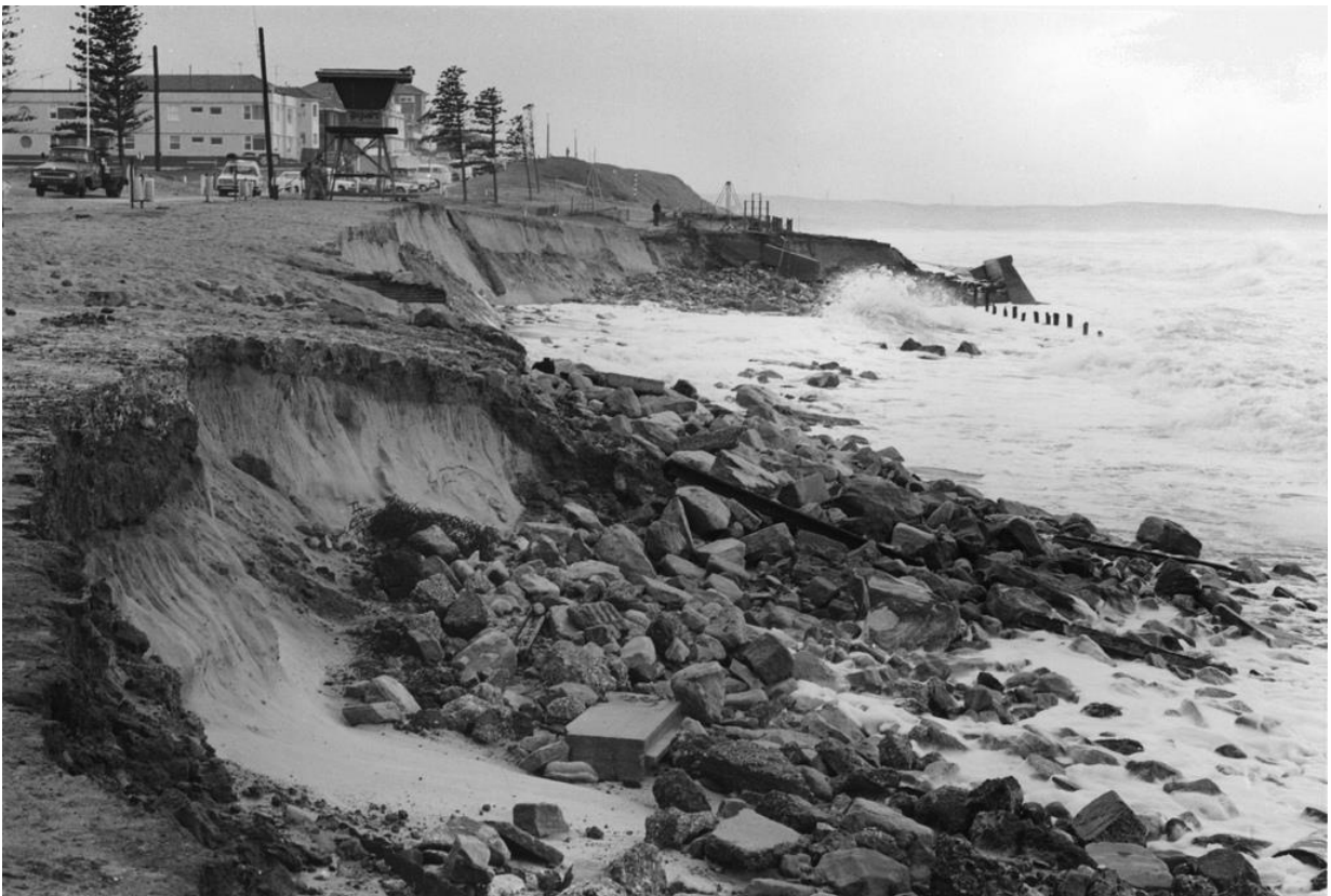
Figure 8-13: 1974 Storm Erosion at North Cronulla Beach
