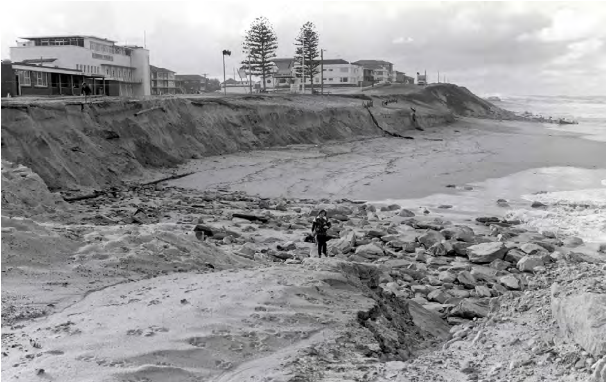
Figure 8-12: 1974 Storm Erosion at Dunningham Park
