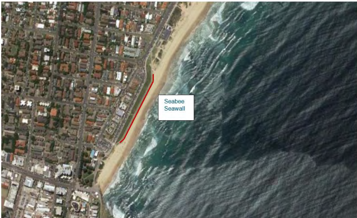
Figure 7-1: Site Location - Aerial View of Prince Street Seabee Seawall, North Cronulla
