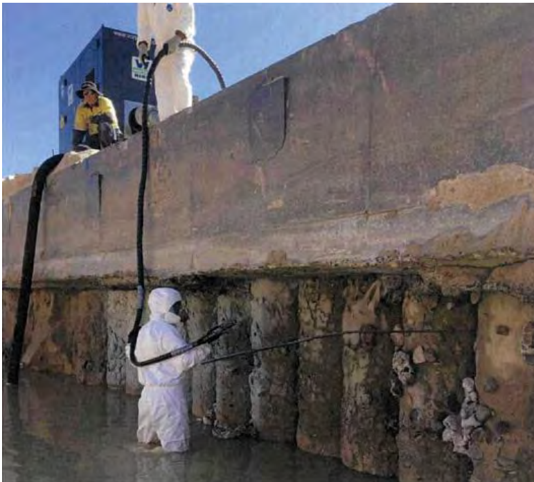
Figure 7-3: Trial Application of Encap-6 to Contiguous Piles
