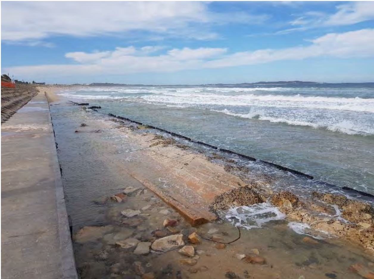
Figure 8-11: Exposed remnants of historical demolition of old seawall
