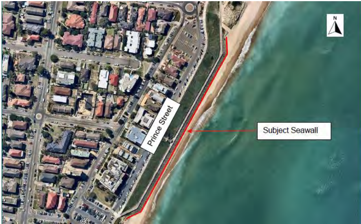
Figure 8-8: Prince Street Seawall
