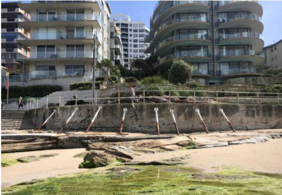
Figure 8-6: Concrete/sandstone block/rendered seawall supporting The Esplanade, northern end of Cronulla Beach
