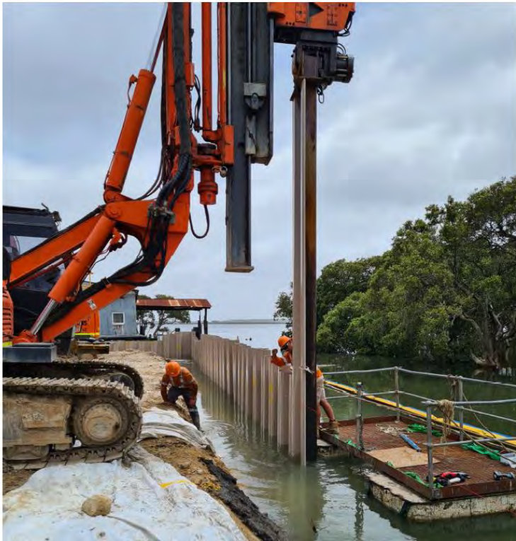
Figure 7-6: Vinyl sheet installation at Woolooware Bay using mandrel (Ford Civil)
