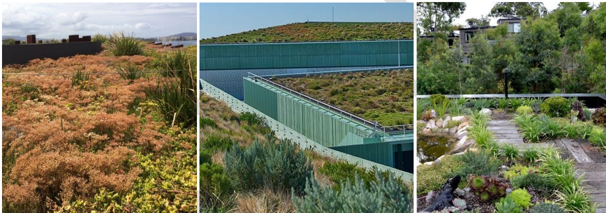
Figures 5.34, 5.35 and 5.36. Extensive green roofs at MONA, Hobart (left), on the Victorian Desalination Plant (middle), and on a residential property in the Sydney central business district (right). Sources: P. Osmond (2016) (left); Aspect Studios (n.d.-b) (middle); Green Roofs Australasia (2014) (right).
