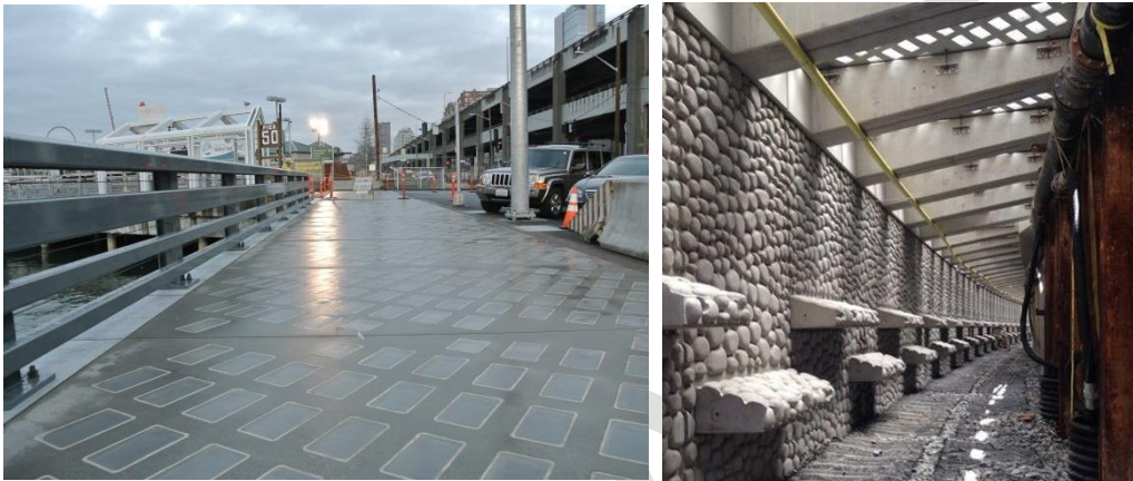
Figures 5.47 and 5.48. The Seattle Waterfront Park pier (left) and seawall (right) are examples of sensitive waterfront designs that have improved coastal ecosystem functioning. Source: Mah (2015).
