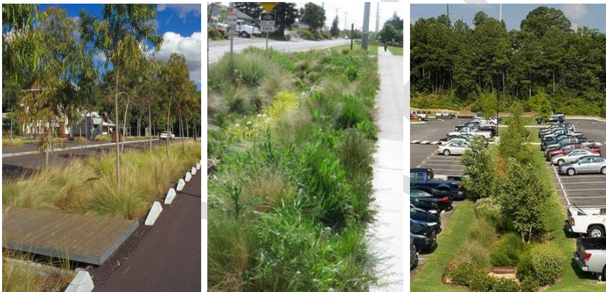
Figures 5.42, 5.43 and 5.44. Bioswales manage urban stormwater flows and reduce pollutant loads, and they have the potential to increase urban biodiversity outcomes when designed appropriately. Source: NSW Government Architect's Office (n.d.) (left); Skoor (n.d.) (middle); All Terrain Consulting Ltd. (n.d.) (right).
