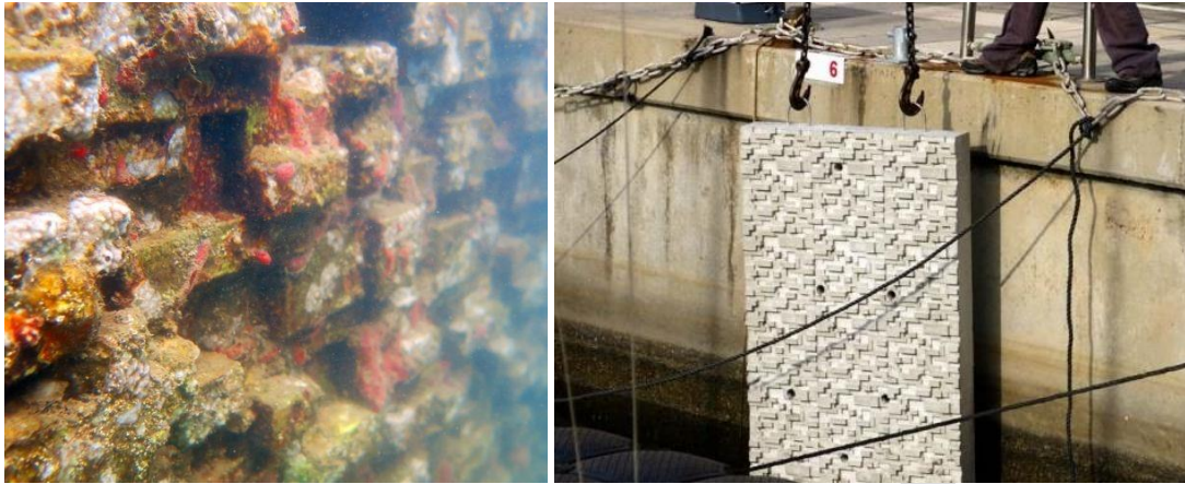
Figures 5.65 and 5.66. EConcrete panels support marine biodiversity. Source: EConcrete (2012).
