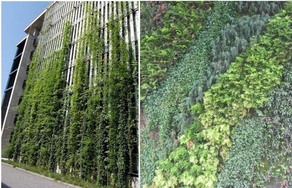
Figures 5.8 and 5.9. The green facade at Sihl City Shopping Centre in Zurich (left) and the living wall at One Central in Sydney (right). Sources: MMA Architectural Systems (2017) (left); P. Osmond (2016) (right).
