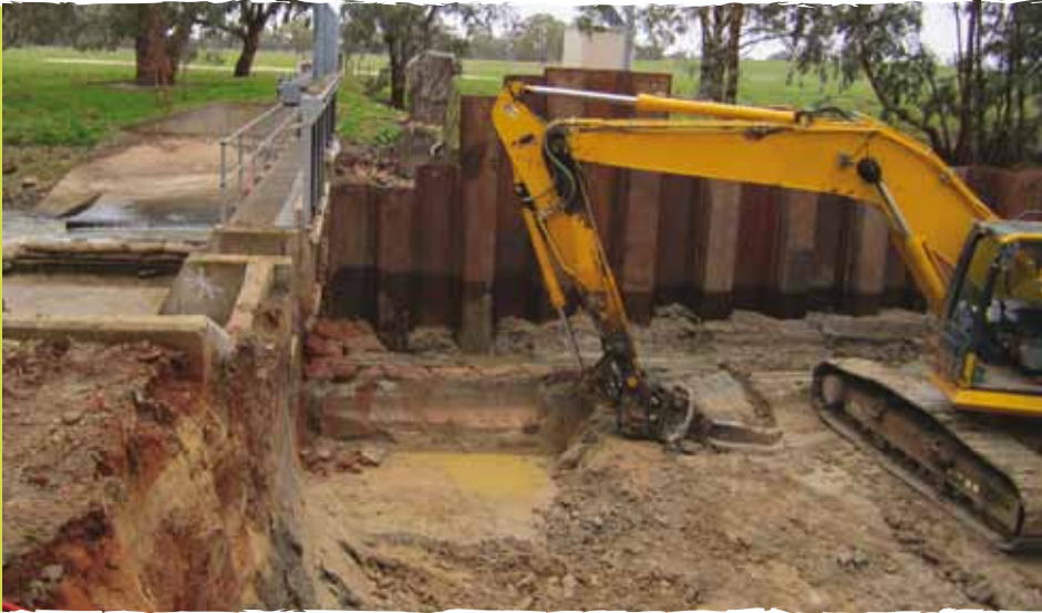
Tarabah Weir Fishway under construction, July 2010.
