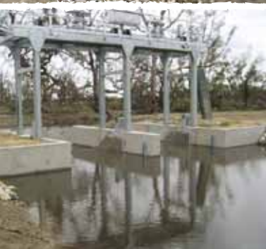
The completed Muggabah Regulator, August 2010.
