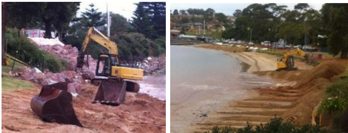
Figure 2-5 Revetment repair works (left) and beach scraping (right), after the June 2016 ECL. Image source: SCC.
