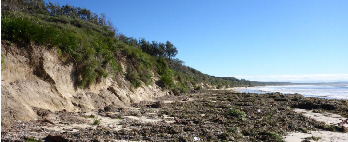
Figure 2-4 Erosion at Currarong Beach after June 2016 ECL. Image source: DCCEEW.
