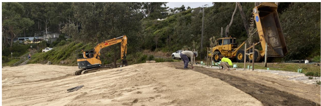
Figure 2-9 Beach scraping and dune rebuilding works undertaken by Council at Narrawallee Beach in June 2022. Image source: SCC
