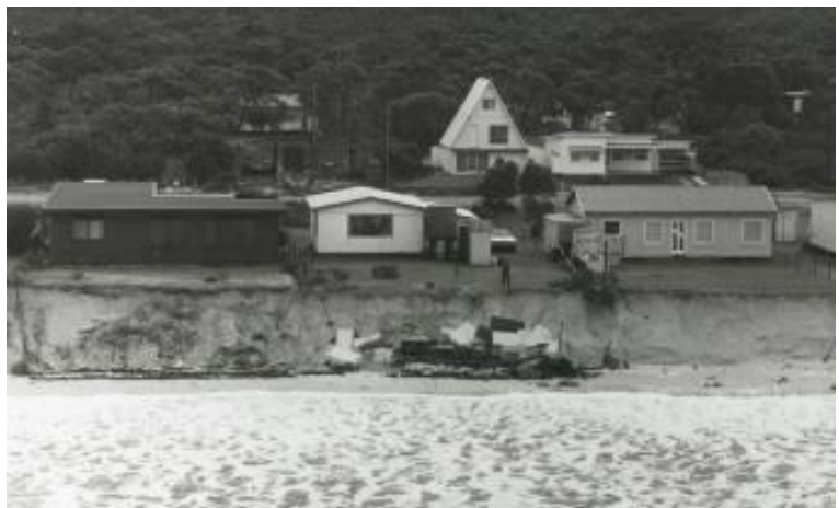
Figure 2-3 The Callala Beach coastal erosion event of 1974. Image source: A. Gordon
