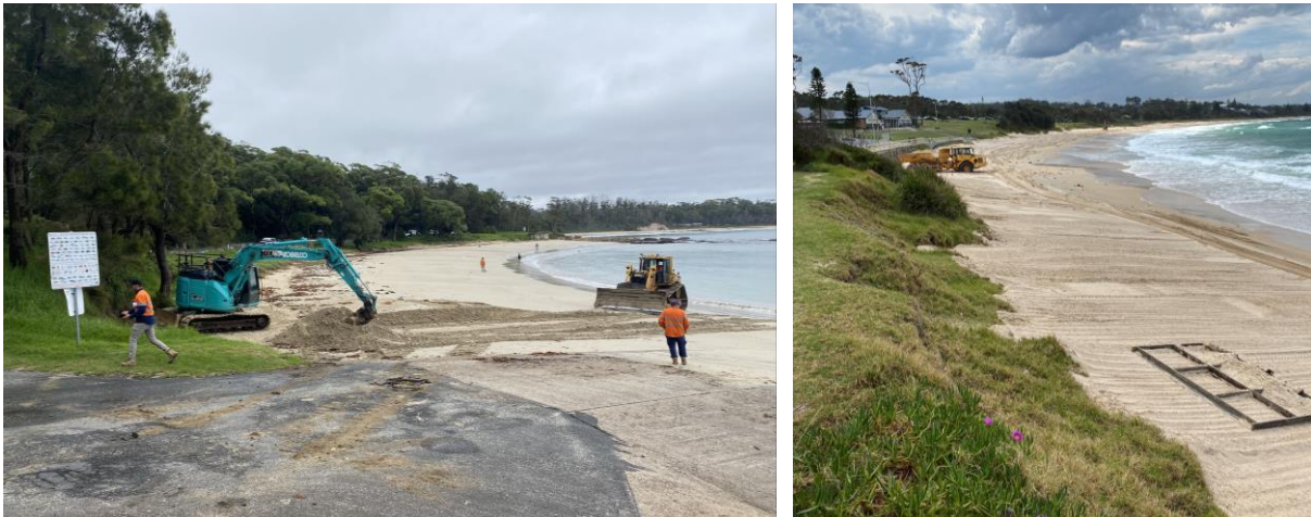
Figure C-1 Emergency beach scraping works undertaken by Council after storm events. Left: Bendalong Boat Harbour, April 2022. Right: Mollymook Beach, June 2020. Image source: SCC
