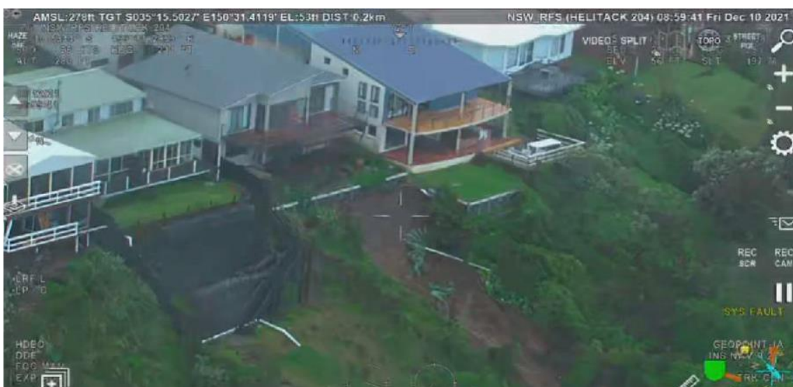
Figure 2-11 Coastal cliff and slope instability event at Inyadda Point following heavy rainfall in December 2021. (Douglas Partners, 2023)
