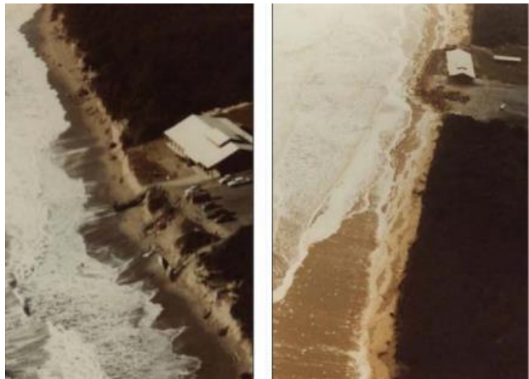
Figure 2-2 Shoalhaven Heads Beach showing Surf Club in 1977 (left) and following rock protection in 1978 (right). Image source: DCCEEW.
