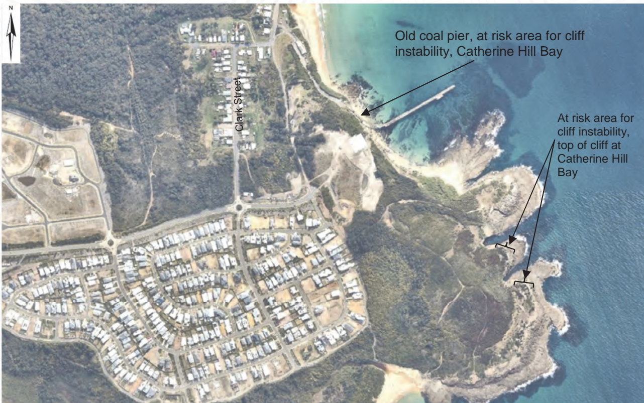
Figure 10: Location of risk area for cliff instability at Catherine Hill Bay.
