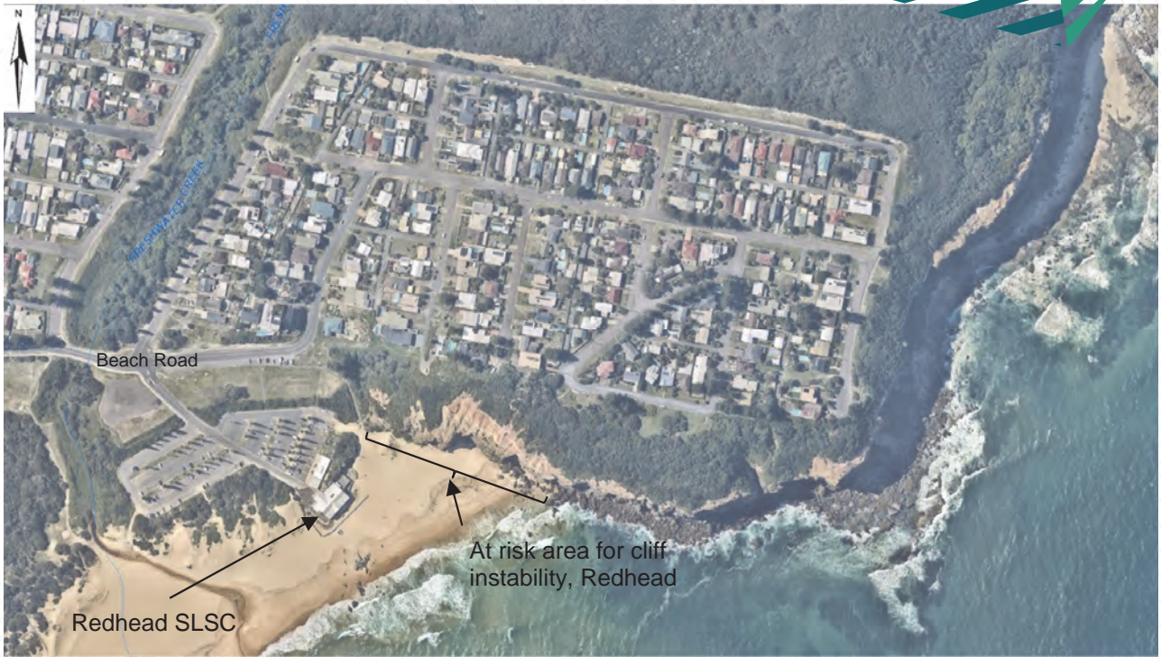
Figure 7: Location of risk area for cliff instability at Redhead.
