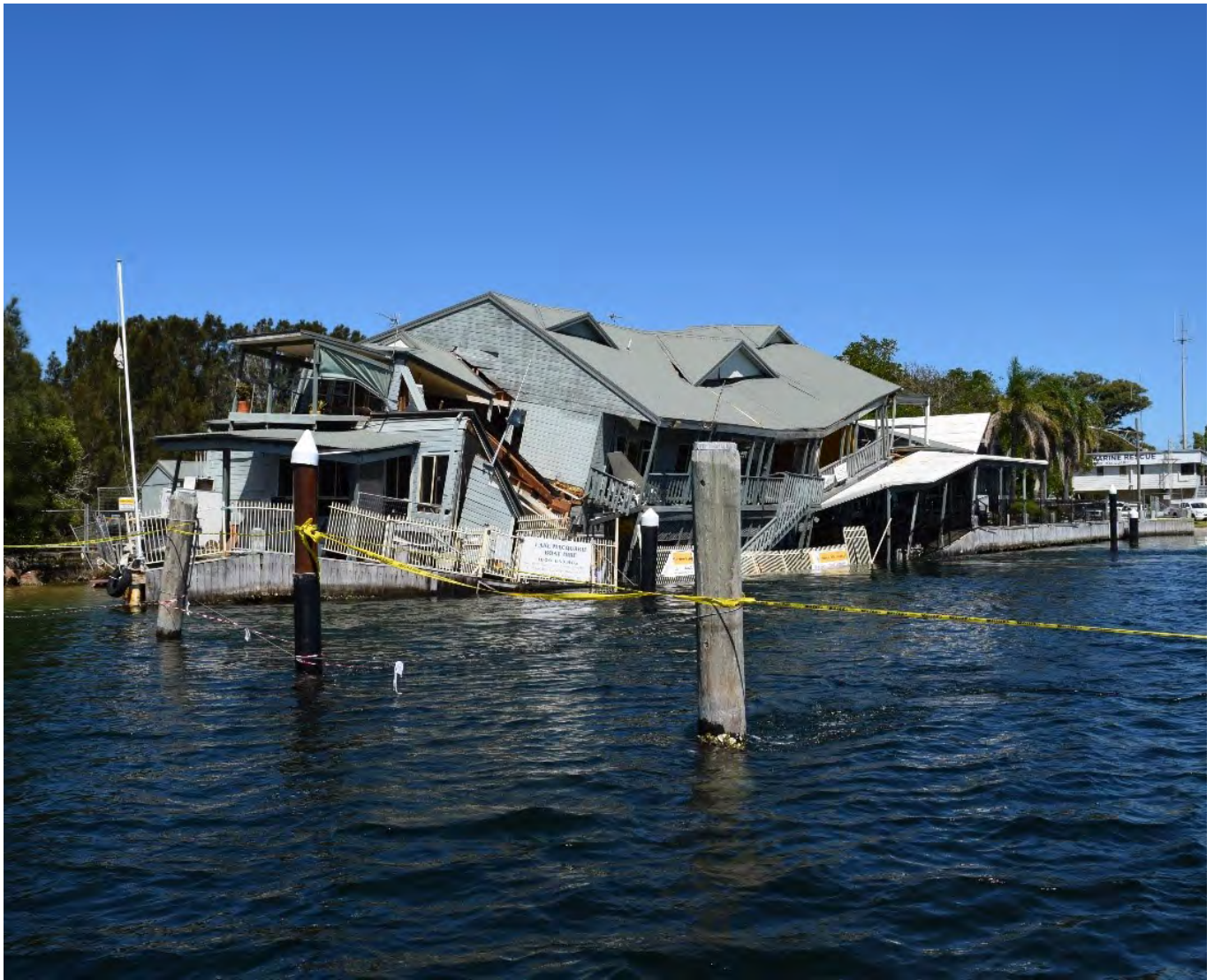
Figure 16: Collapse of Pelican marina complex - February 2016 (Source: S Walpole)
