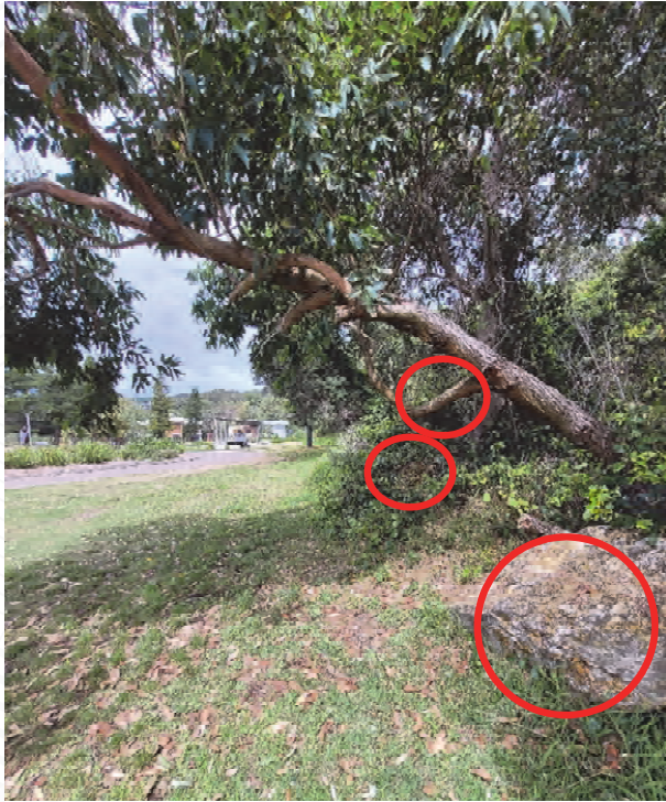
Photograph 5: Caves Beach picnic area, example of historic conglomerate boulder rockfalls (up to ~5m diameter) photographed January 2021.
