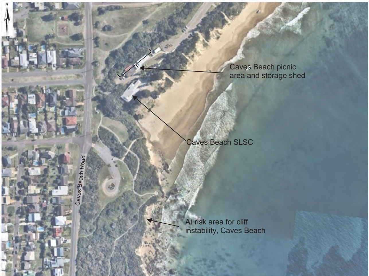
Figure 8: Location of risk area for cliff instability at Caves Beach.
