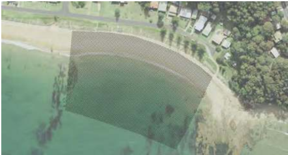
Figure 2 Long Beach Sand Nourishment
