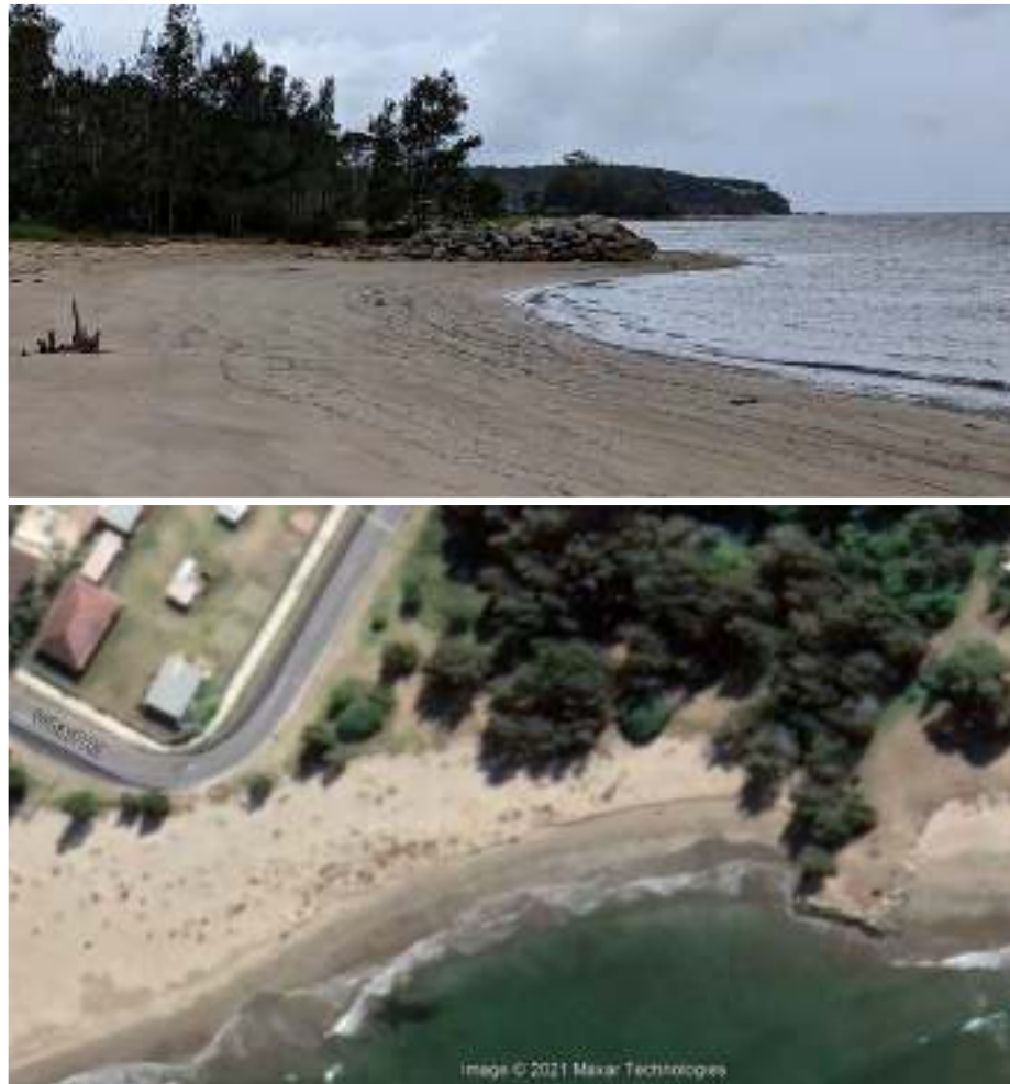
Figure 5. Photo and location of unapproved coastal protection structure at the Wharf Road subdivision.
