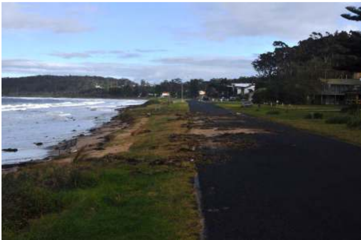
Overtopping of Bay Road, Long Beach, 6 June 2012 (Mr Lindsay Usher) – from WRL, 2017
