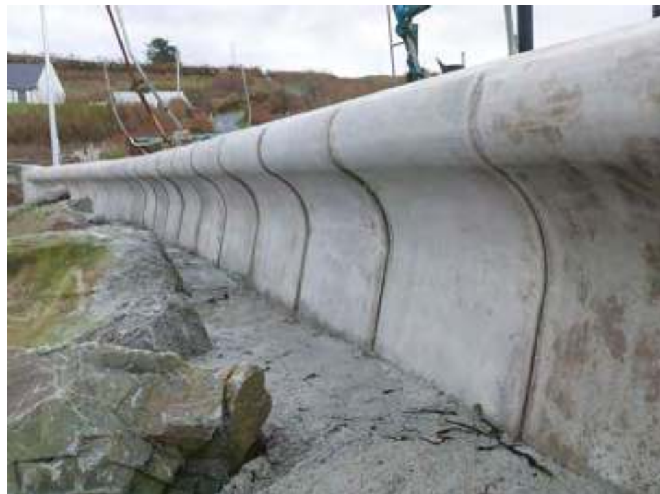
Figure 7 Example of a concrete wall return barrier
