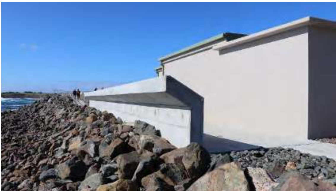
Figure 2 Example of wave return barrier, Port Kembla (from MHL, 2021)
