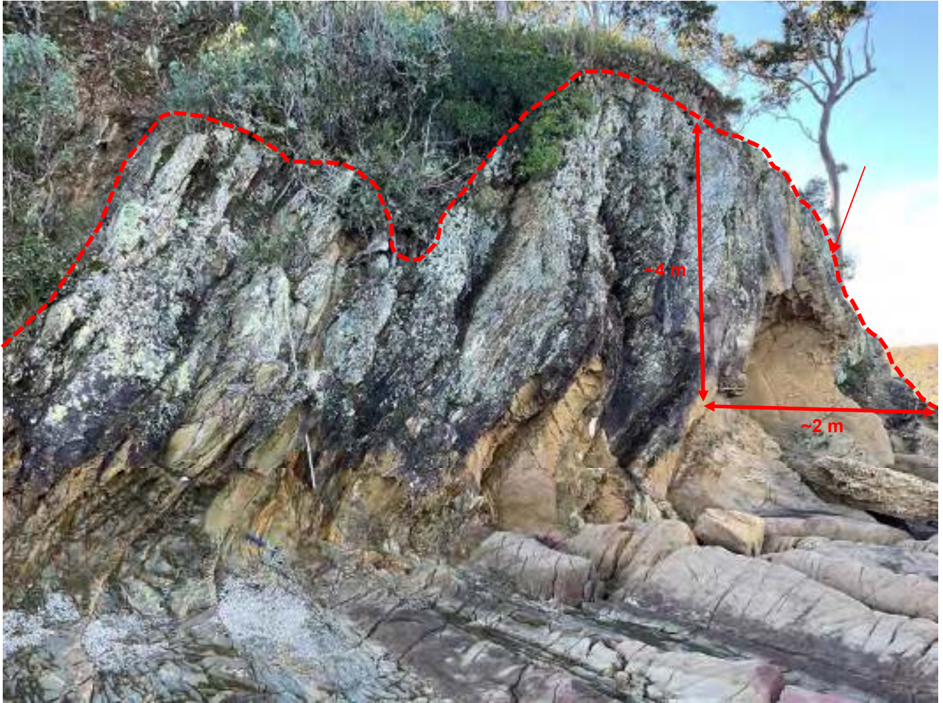
Inset 5: Example of variability in the bedrock:soil interface (~4 m vertical drop over ~2 m horizontal) identified during the mapping campaign. In this example at Surfside North, the variable rock:soil interface is controlled by bedding structure in the rock.
